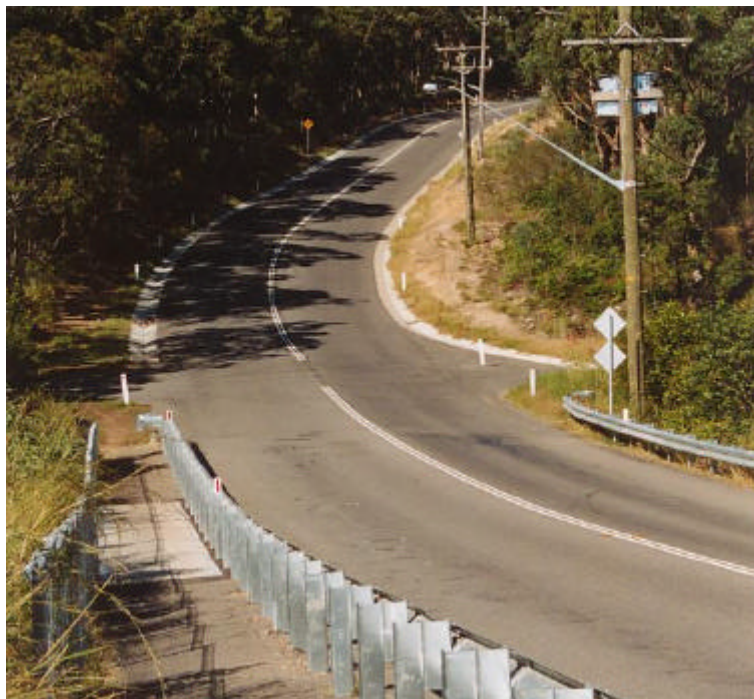
A 1 km section at the northern end of Burwood Road Whitebridge was rebuilt by Lake Macquarie City Council during 2002, adjoining the newly completed Fernleigh Track. Apart from a short section across Flaggy Creek, the new road work contains no provision for pedestrians or cyclists, even though this is a popular area for walking and cycling, and there was ample width to include a separate pathway.
