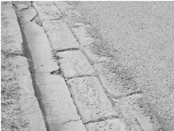
Example of bitumen extending over the sandstone kerb and guttering
