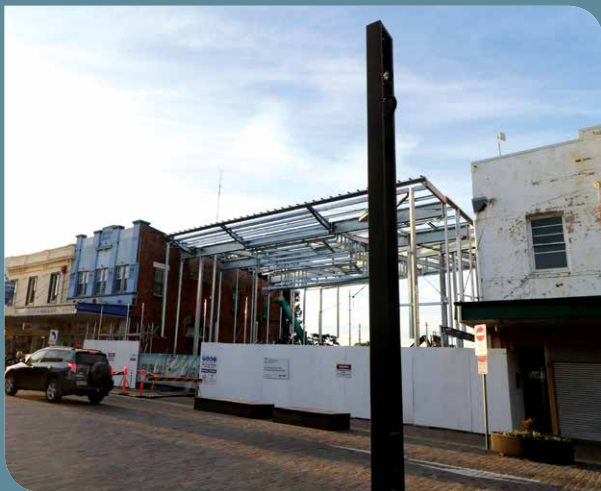
Progression of The Levee Riverlink Building continues
