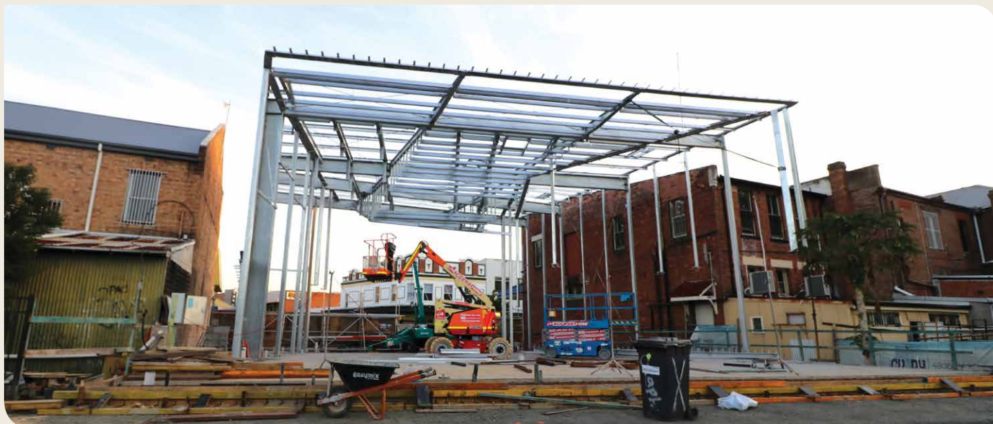
Construction of The Riverlink Building is progressing well at The Levee
