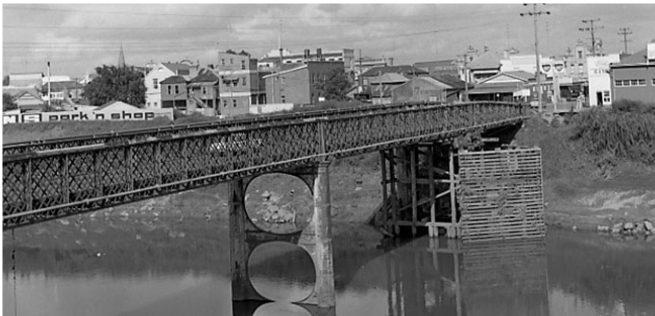
Figure 4.1: Belmore Bridge before being replaced by the current bridge.
