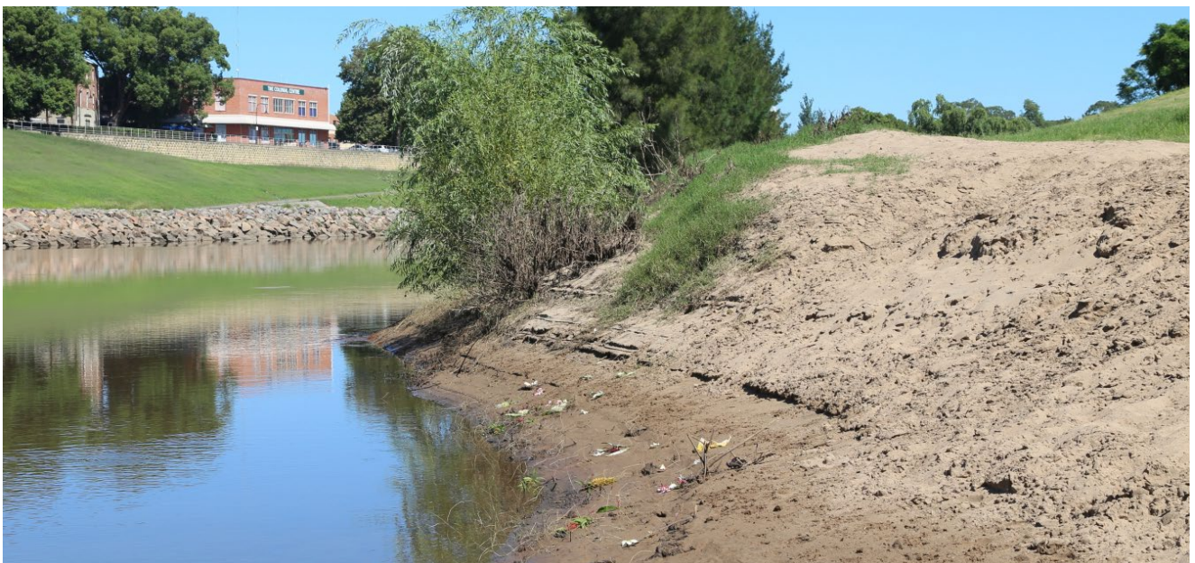
Figure 7.3: Sandy banks rising steeply from the river stabilised by vegetation.
