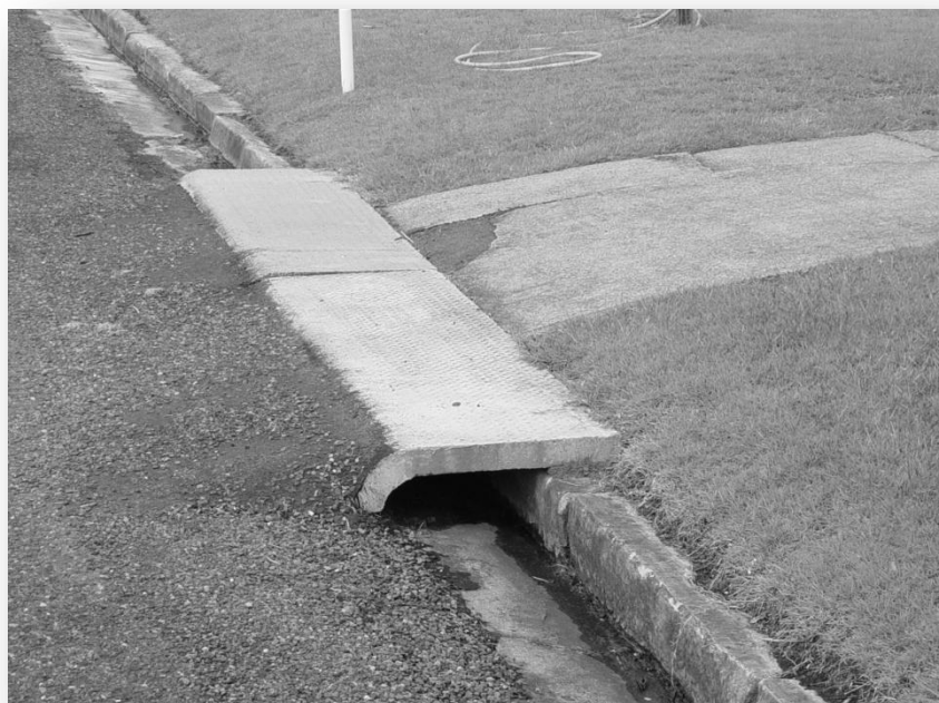
Example of a new kerb bridge
