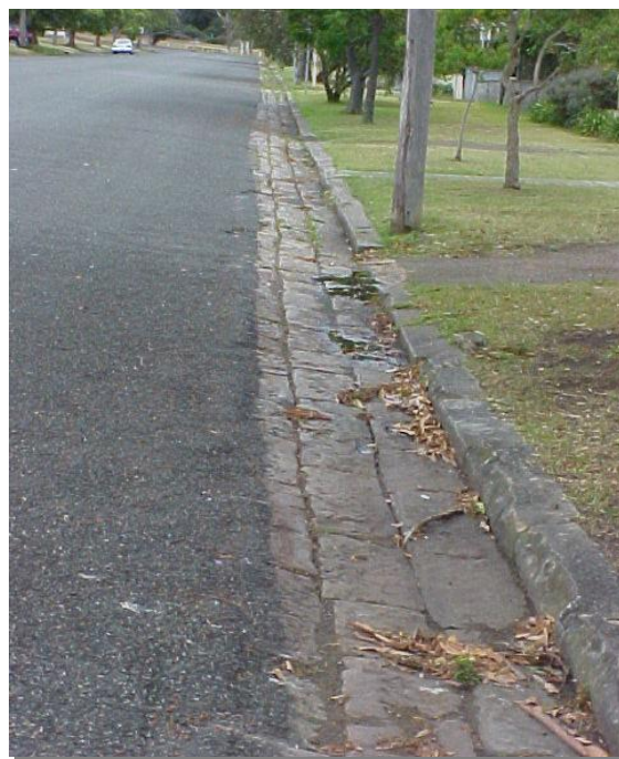
Sandstone Kerb and Guttering in High Street
