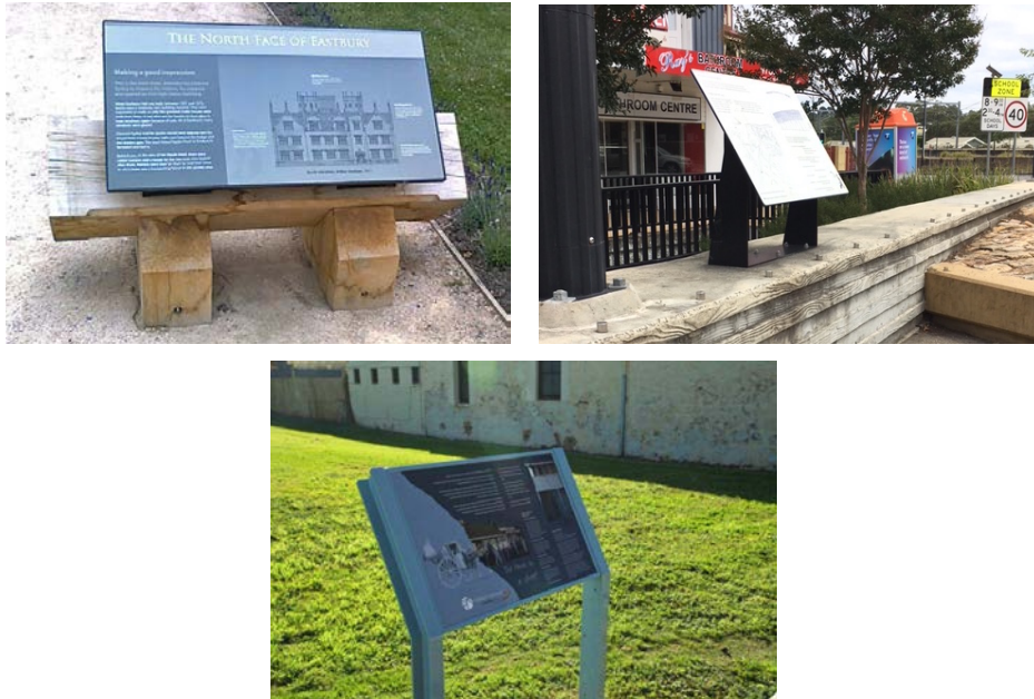
Figures 7.2.6e, f, g: Gary Luke located these images on the web and thought the mounting methods of interest. ‘Rough blocks of timber. The bent metal legs. A folded sheet metal support. The same structural forms could be used for a seat. I picked them also because of their proportions - wider than high.’ 153
