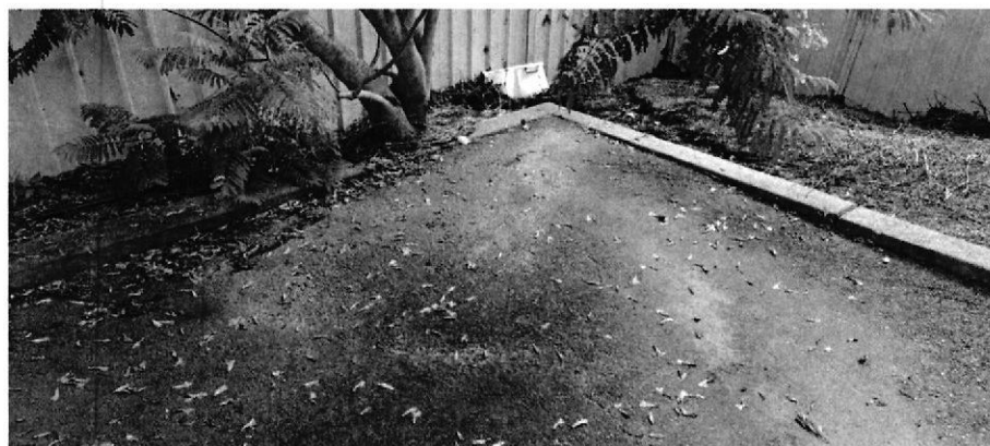
Photo 2 – The tar in the childcare centre carpark comes up to the top of the kerb and gutter (in dry conditions)
