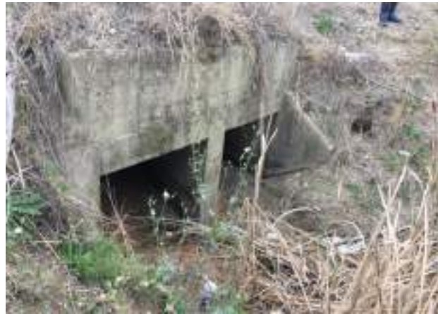
Photo 9 – Road Culverts underneath Northcote St, Kurri Kurri
