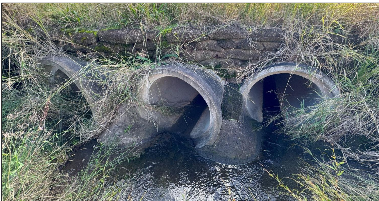
Figure 18. Three pipe-culvert in the south of the Subject Land.
