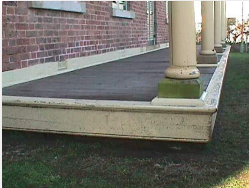
Wooden items need regular maintenance and should be inspected every six months
