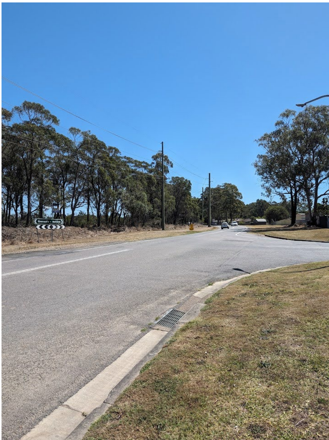
Haussman Drive and Talyor Avenue Intersection looking north along Haussman Drive - on left hand side some of the vegetation will require removal and electrical infrastructure will require relocation
