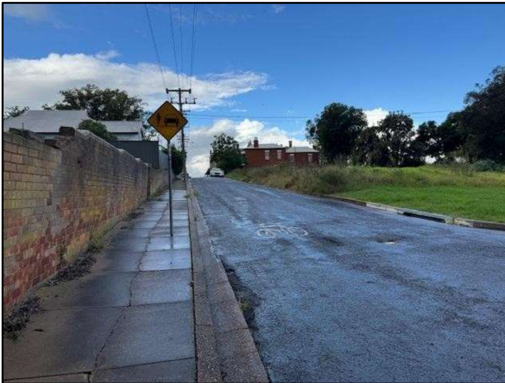
Photo 1 – Visibility looking east along Steam Street showing cross section and on road cycling
