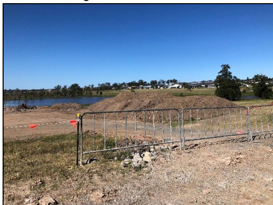
Photo 7: View at site frontage looking northeast at the east side temporary access point.
