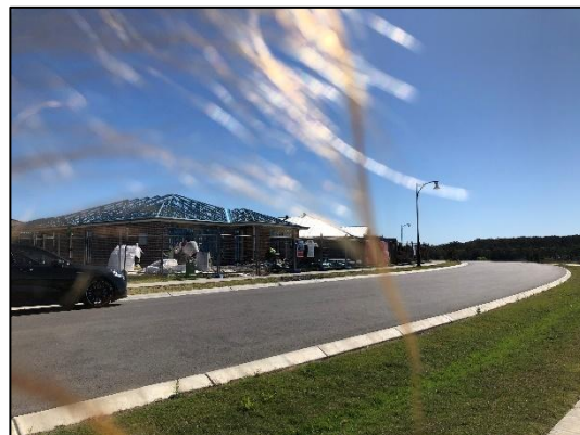
Photo 6: View at site frontage looking south at no. 75 Billabong Parade.
