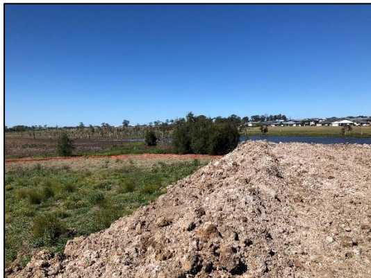
Photo 17: View at northeast side of fill mound looking north towards waterway
