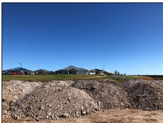
Photo 19: View at west side of fill mound looking south towards Billabong Parade.
