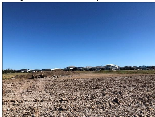
Photo 16: View at northeast side of fill mound looking south towards Billabong Parade.
