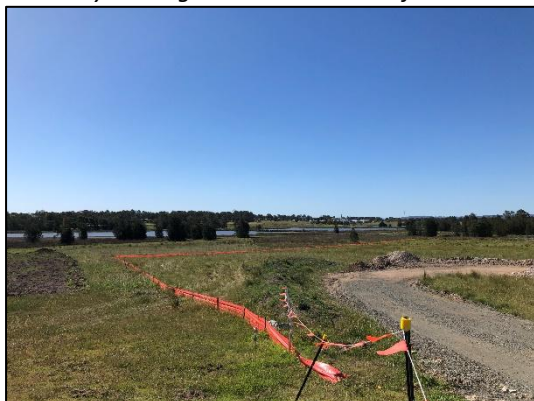
Photo 23: View from Billabong Parade at the west side temporary access point looking north.
