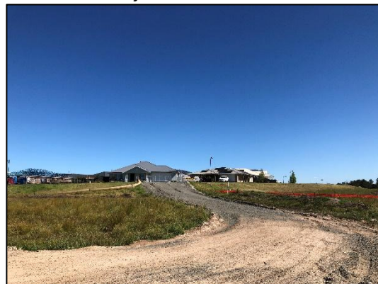
Photo 22: View at west side of fill mound looking south towards Billabong Parade/access point.
