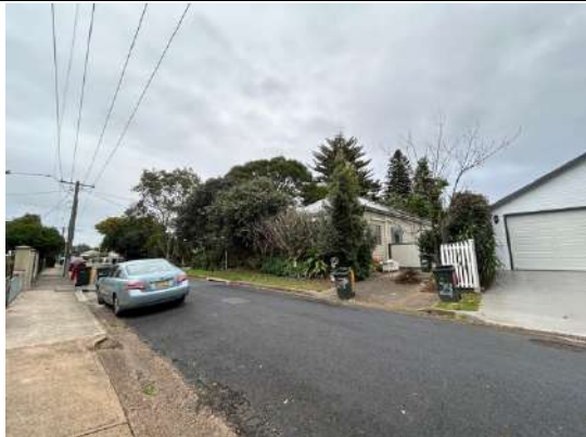
Looking from the front boundary across James Street in a south westerly direction.
