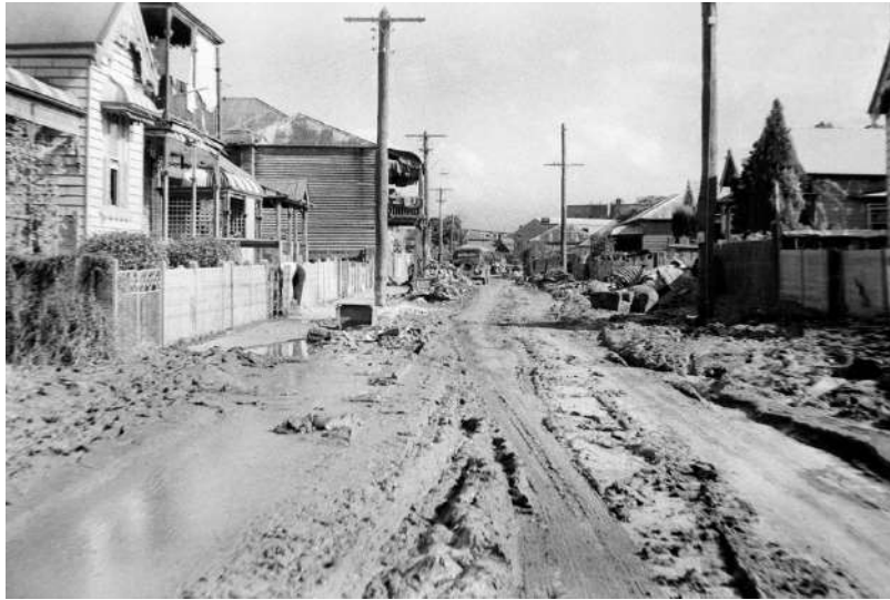
Figure 27 Maitland Flood Damage, 1955: Lucy Collection.
