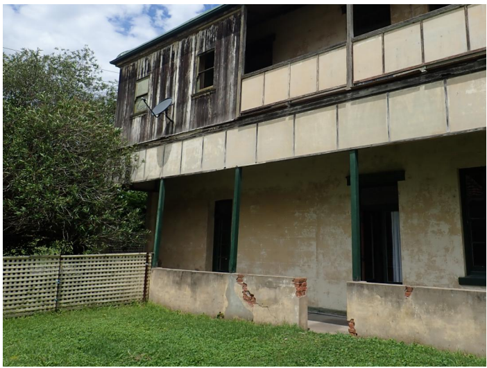
Photograph 6. North facade. Heavily modified. Asbestos panels and veranda infill.
