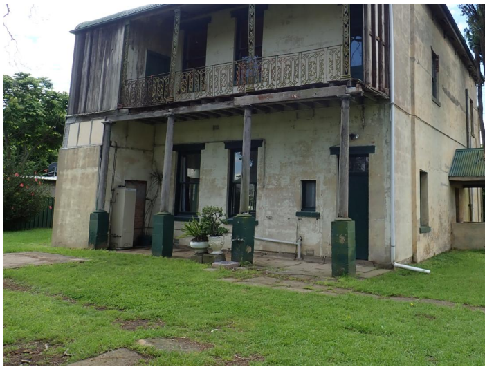
Photograph 5. West facade. Heavily modified, however existing ornate balustrade and columns remain.
