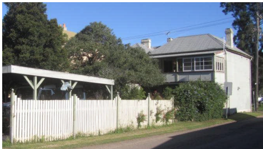
Plate 11: The rear verandah appears to have been enlarged. (JCHD 9280)
