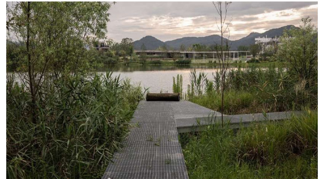
Example of elevated boardwalk around filter beds
