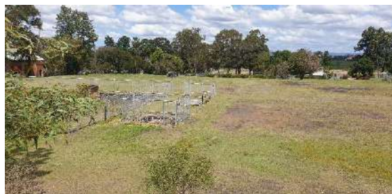
Figure 15: View south, showing overall view of tanks, beds and basin located west of the pumphouse
