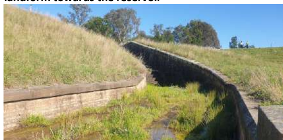
Figure 19: View north, showing the brickwork reservoir spillway
