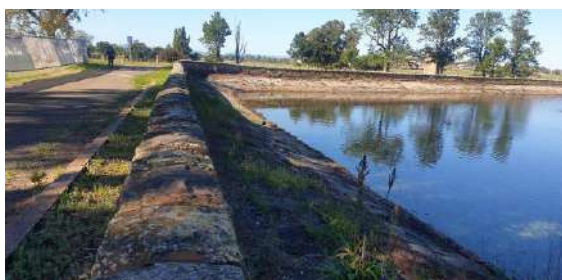
Figure 13: View south within walking trail on perimeter of reservoir
