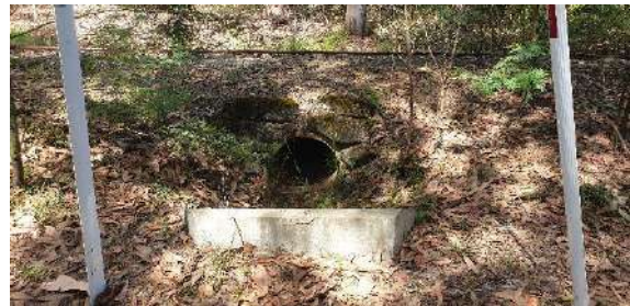
Figure 27: Drainage culvert constructed below walking trail
