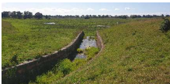
Figure 23: View south, from the top of the spillway
