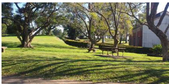
Figure 11: View north from the main access road, showing landscaping and battering surrounding the western portion of the pumphouse
