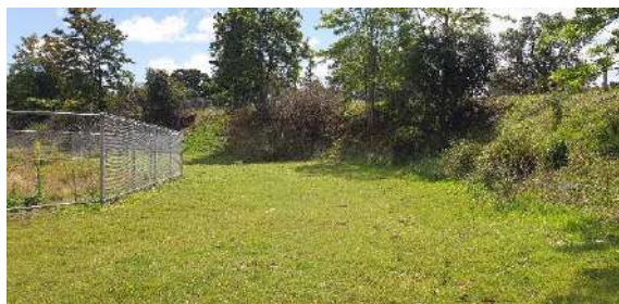
Figure 14: View west next to filter bed, showing battering
