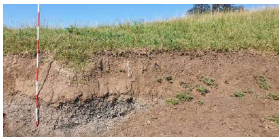
Figure 18: Exposure identified near the spillway, showing homogenous brown clay loam, with a pocket of gravel fill
