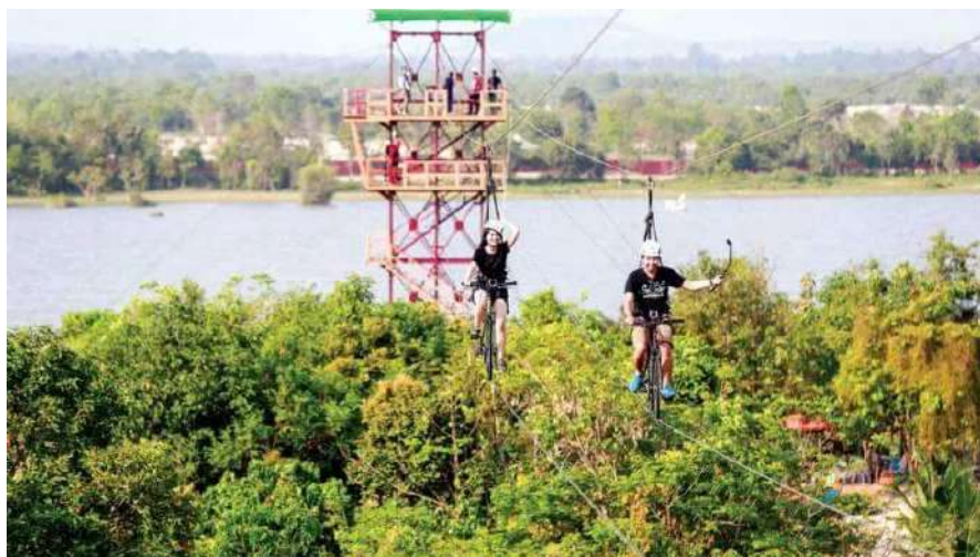
Figure 2.7.2 Example of sky cycling and supporting towers
