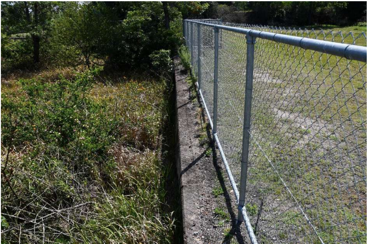
Figure 106: The northern wall of Filter Bed 6 (Item J-6) with the concrete coping evident. View to the west
