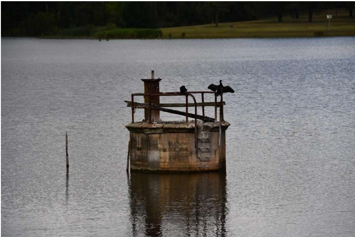
Figure 129: The outlet tower within the eastern end of the Reservoir. View to the East
