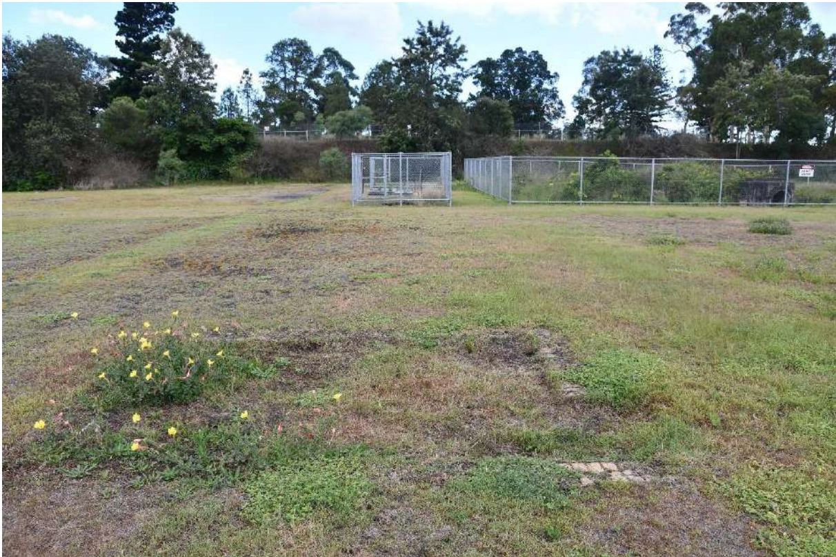
Figure 116: The southern access point where only the upper course of bricks remains visible. View to the north
