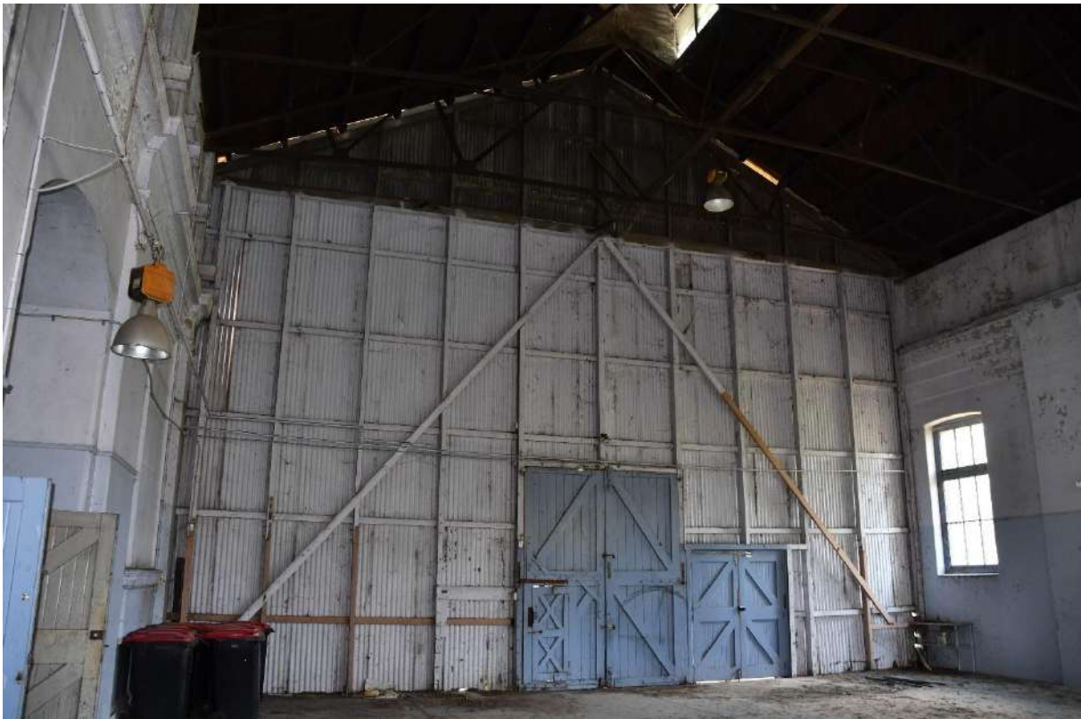
Figure 76: The internal side of the southern elevation of the Western Pumphouse (Item F) demonstrating the timber frame to which the iron cladding is attached. View to the south
