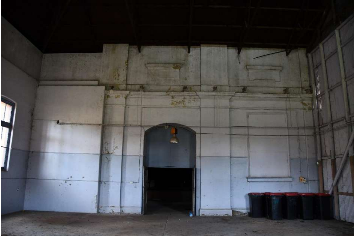
Figure 77: The internal eastern wall of the Western Pumphouse (Item F) showing the doorway through into the Main Pumphouse (Item A). Features from the originally external western wall of the Main Pumphouse are clearly visible. View to the east.
