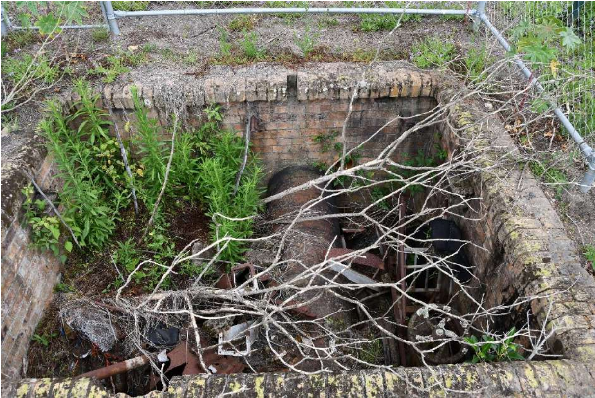
Figure 118: The intact northern most access point where the brick work, main pipe and numerous other fixtures and fittings are visible. View to the north.
