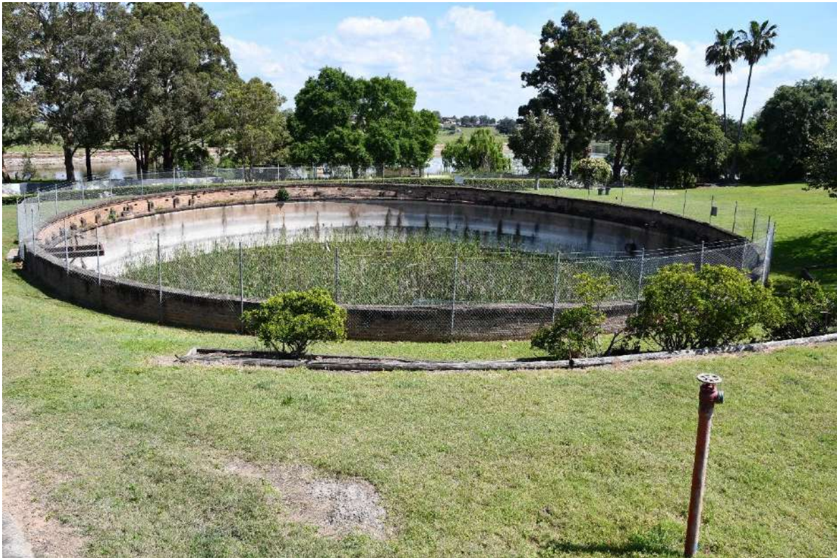
Figure 111: General view of the Clear Water Tank facing south. The gated inlet area is visible as are a number of the internal roof pillars.
