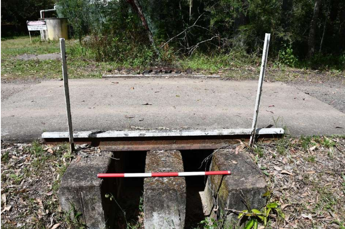
Figure 92: One of the small bridges seen along the route of the former railway. Here it appears the c.1950s concrete bridge structure was modified to carry a concrete slab, hemmed with former railway sleepers.
