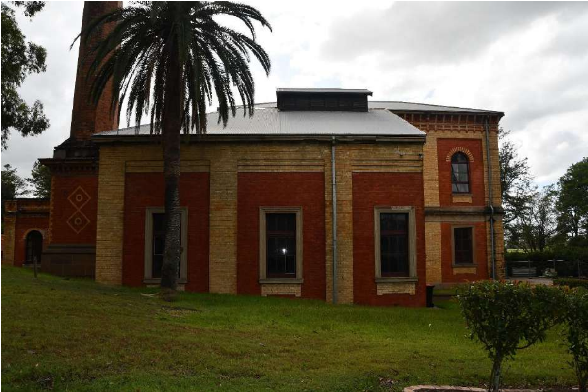
Figure 75: The eastern elevation of the Western Pumphouse (item F). The design and structure of the Western Pumphouse closely match the original Main Pumphouse (Item A) but is less ornate. View to the east
