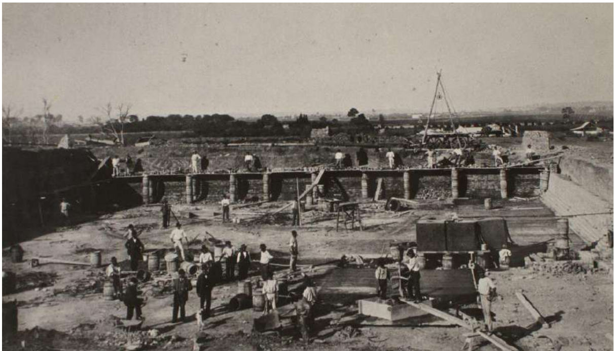
Figure 10: Construction of the Settling tank c.1885. Note the recognisable stepped brick work on the right of the image. Photo from the Maitland City Library Collection
