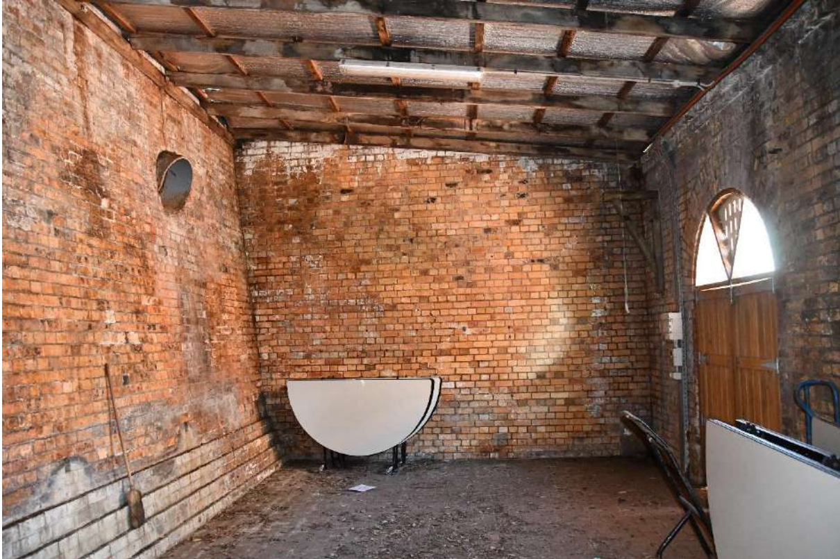
Figure 72: Internal view within Item E facing the eastern wall. The chute for coal delivery can be seen in the northern wall on the left of the image.
