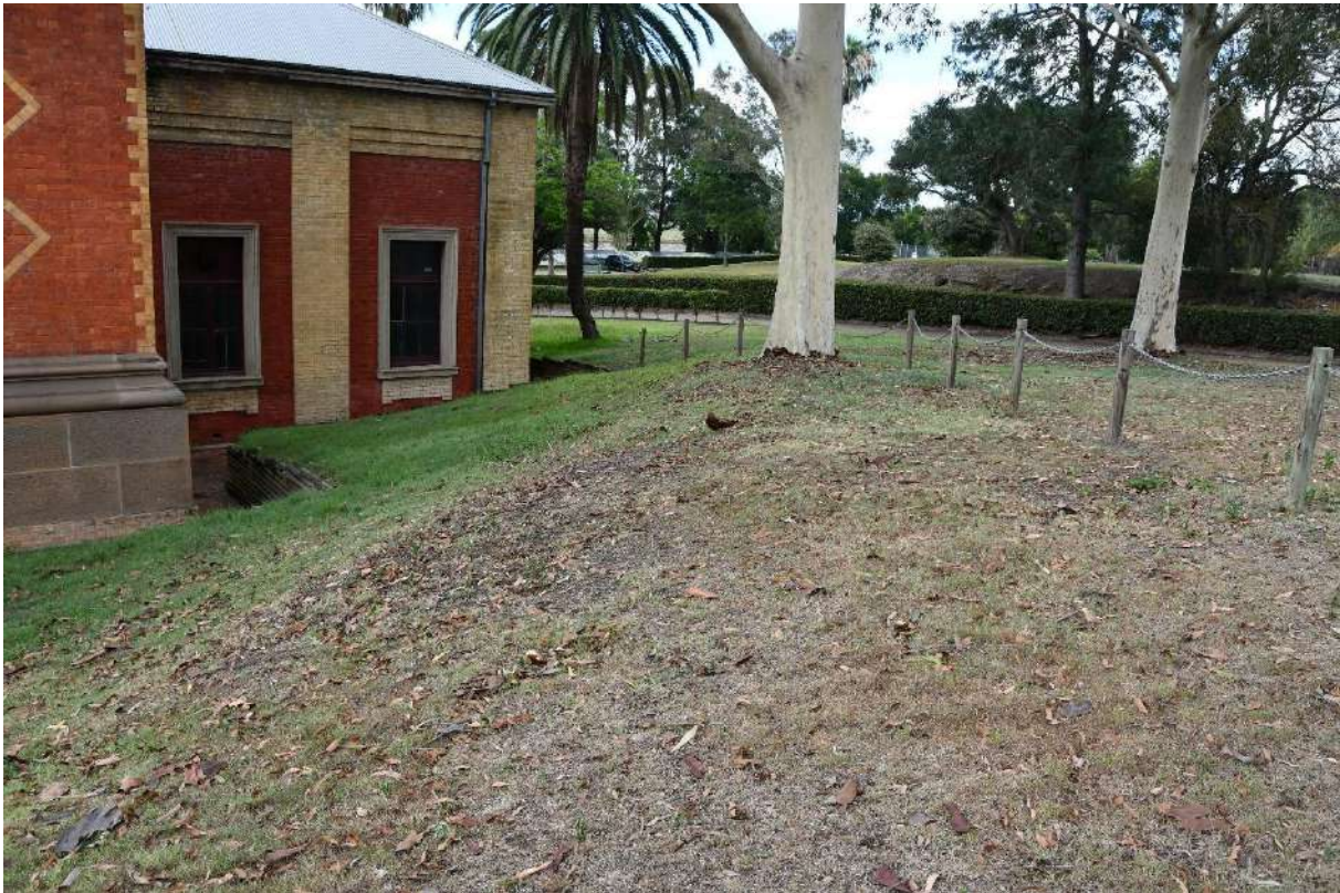
Figure 81: The approximate location of Pumphouse No 6 (Item R) to the north of the chimney (Item C). Evidence of the landscape modifications made during the 1990s can be seen around the chimney (Item C) and Western Pumphouse (Item F) View to the southwest
