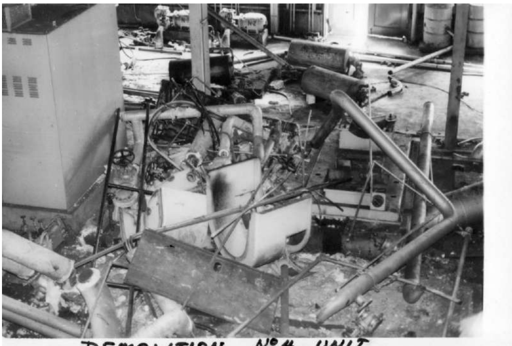
Figure 25: Part of the demolition of the Power Station in 1978 showing the destroyed machinery. Photo provided by MCC.
