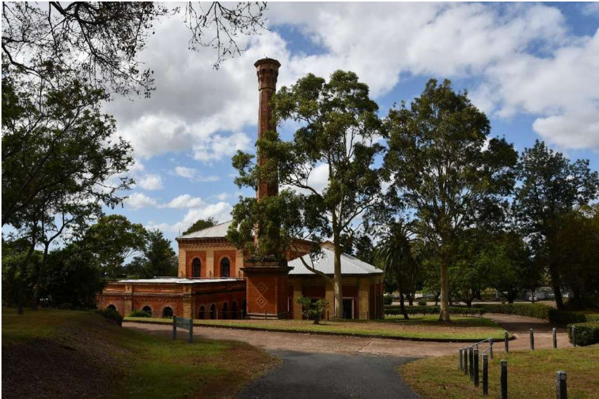
Figure 64: The chimney (item C) viewed from the north showing its location to the west of the Boiler Room (Item B)
