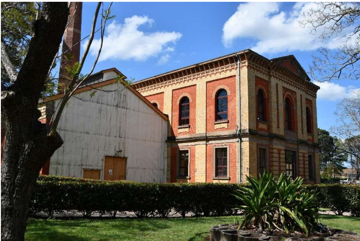
Figure 39: Southern and western elevation of the Main Pumphouse (Item A)
