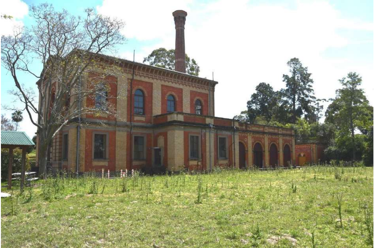
Figure 67: The Eastern elevation of the Pumping Station showing the location and features of the Eastern Annex (Item D). The unsympathetic 1950s doorway is visible on the southern facade of the annex.
