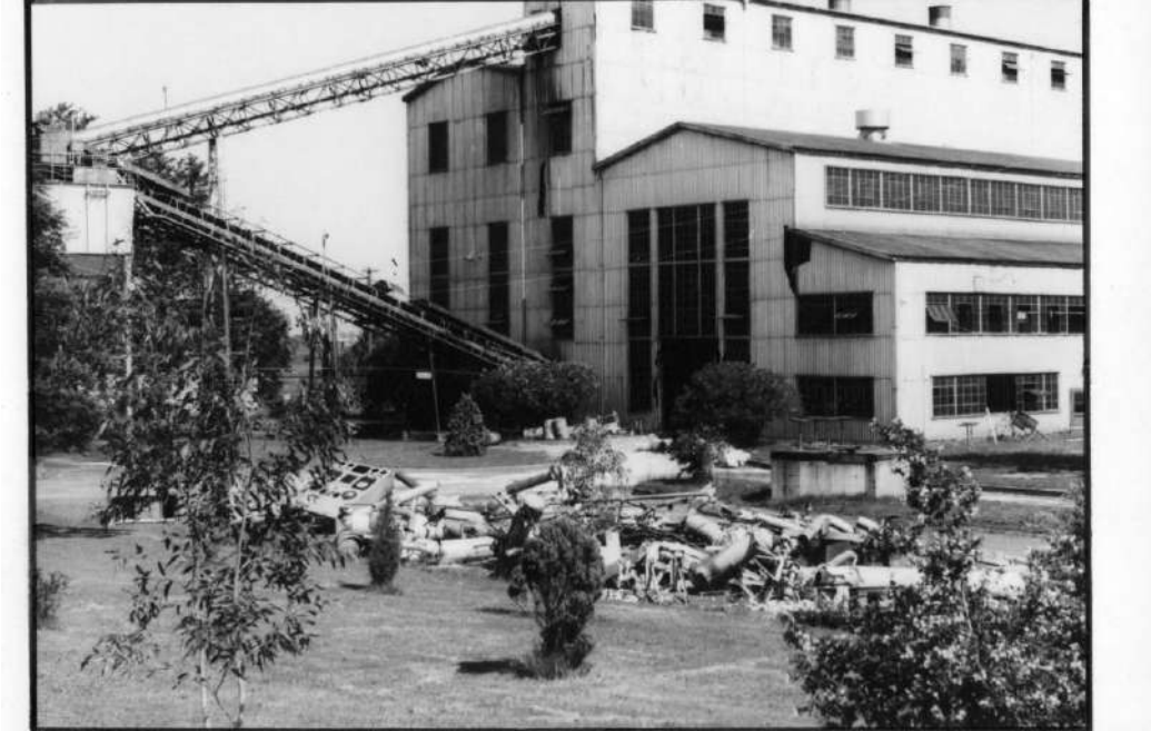
Figure 24: Piles of smashed machinery during the demolition of the Power Station in 1978. Photo provided by MCC.
