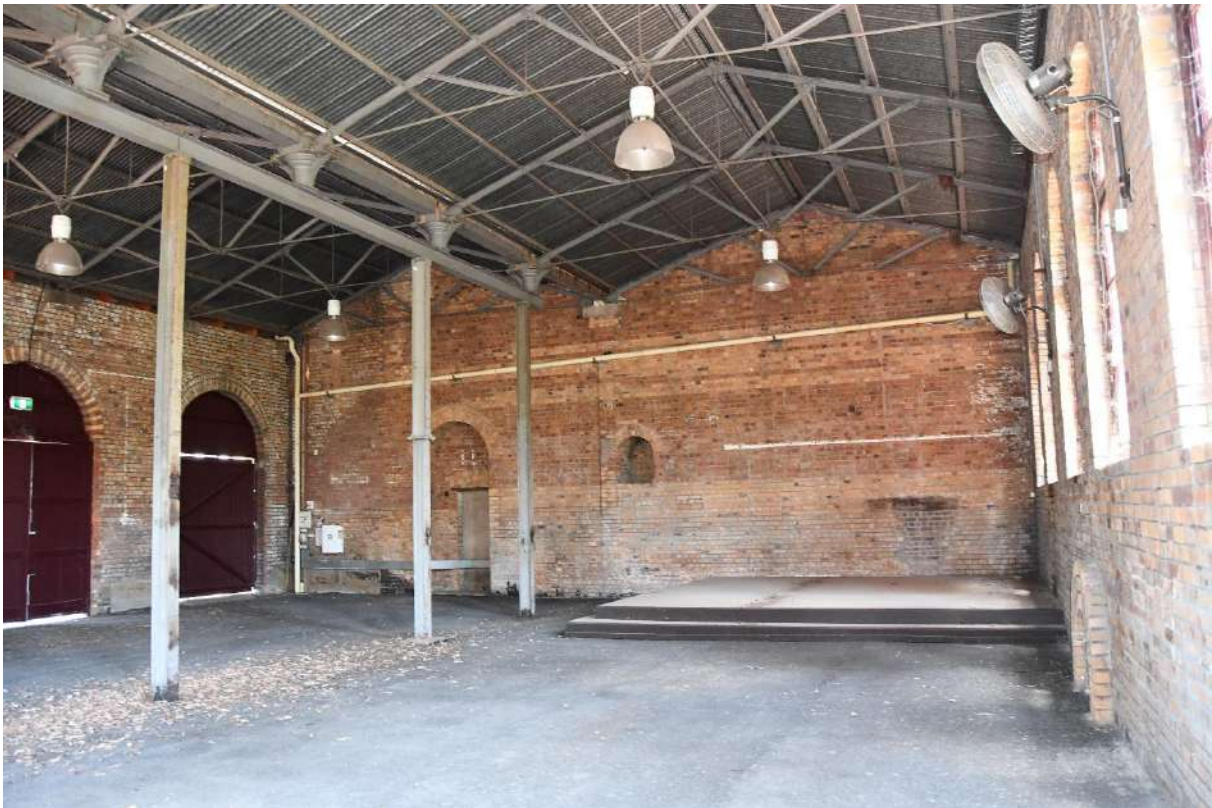
Figure 60: The southern wall of the Boiler Room (Item B) where the various previous access points to the Main Pumphouse (item A) can be seen.
