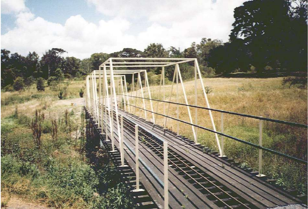
Figure 27: The miniature railway bridge built in 1996 Photo Provided by MCC
