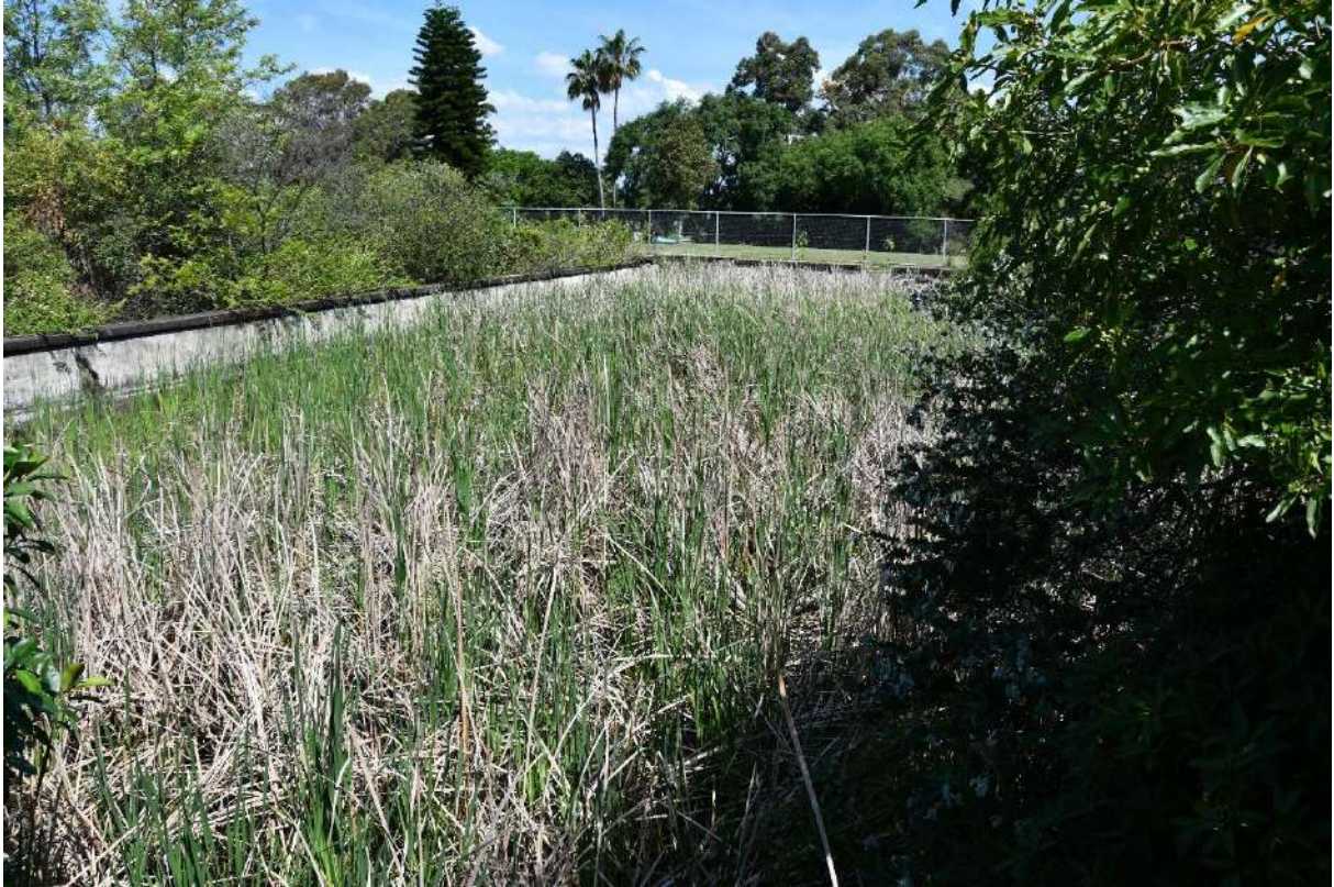
Figure 105: The central wall that divides Filter Bed 5 (Item J-5) and 6 (Item J-6). The intact concrete walls are in good condition however the beds are very overgrown.
