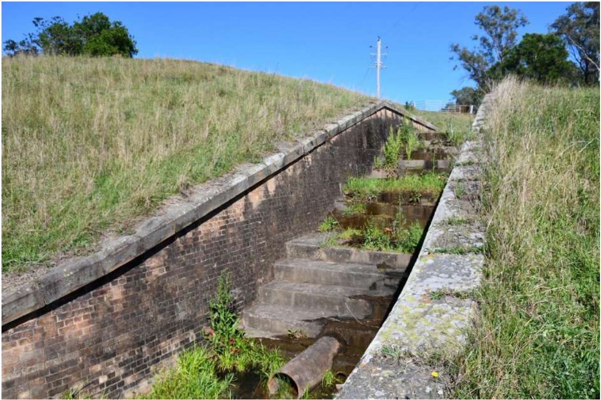
Figure 136: The stepped section of the Byewash showing the outlet from the lower pipe. View to the north.
