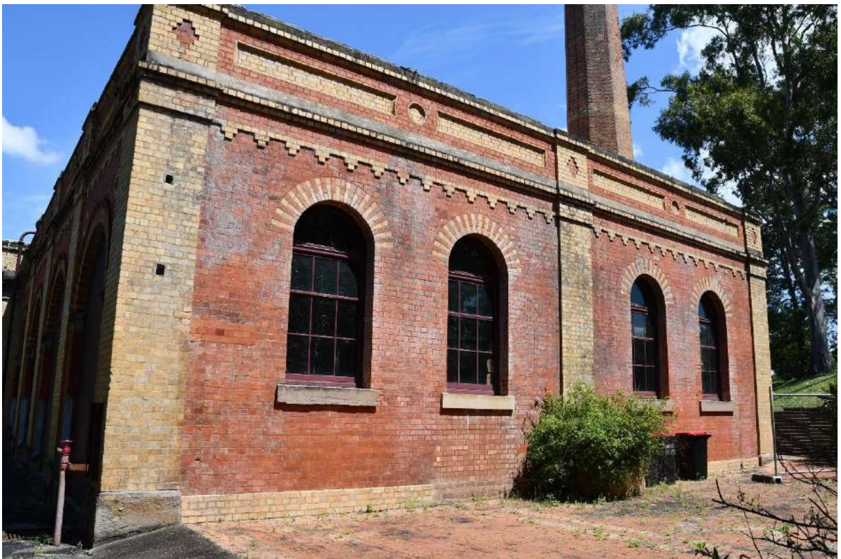
Figure 56: Northern elevation of Boiler Room (Item B). Evidence of the attachment of the former Addition (Item G) can be seen on the corner in the foreground and below the window frame where the brick work has been replaced.
