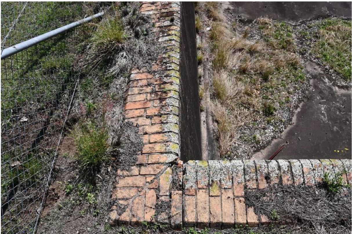
Figure 97: Detail of the northeast corner of the Settling Tank showing the rowlock brickwork on the upper course with mitred corners and cant bricks. View to the south
