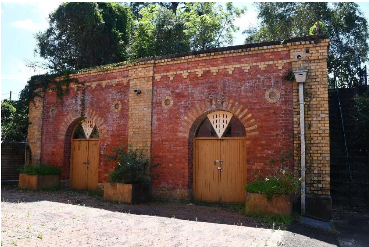
Figure 71: Southern Elevation of the Coal Store / Workshop (Item E). the stairs to the upper street level can be seen on the right of the image.
