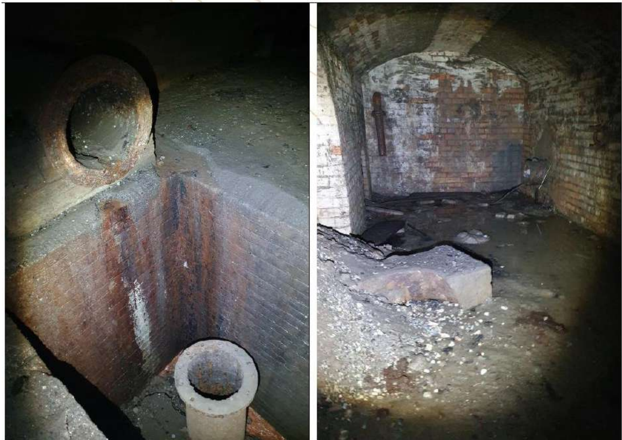
Figure 119: The Western Tunnel that extends out from the Pumping Station with original pipework and potential pump structure remaining. Photo taken by Onyx during the 2020 Exploration on behalf of Maitland City Council.
