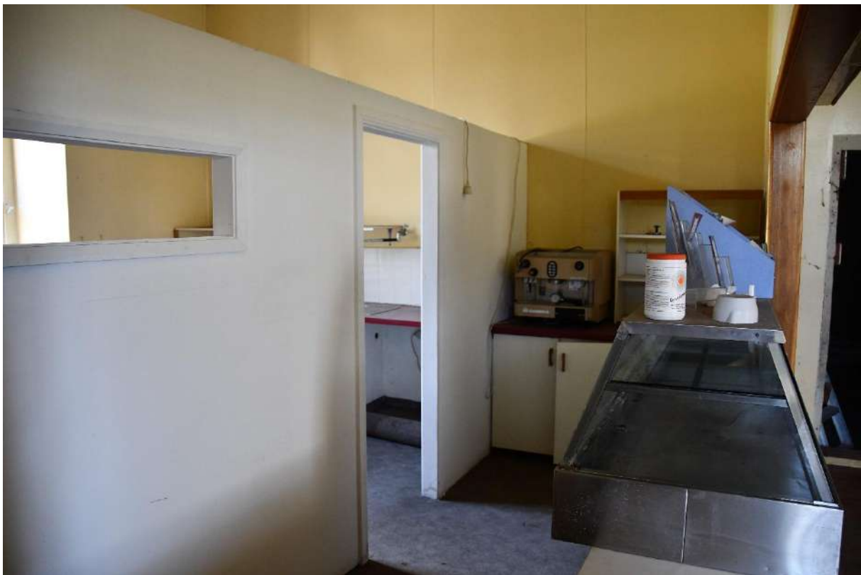
Figure 45: The front section of the Kitchen/Laboratory (Room #03). The low partition wall is of an unknown date but likely was installed along with the kitchen equipment in the 1990s.
