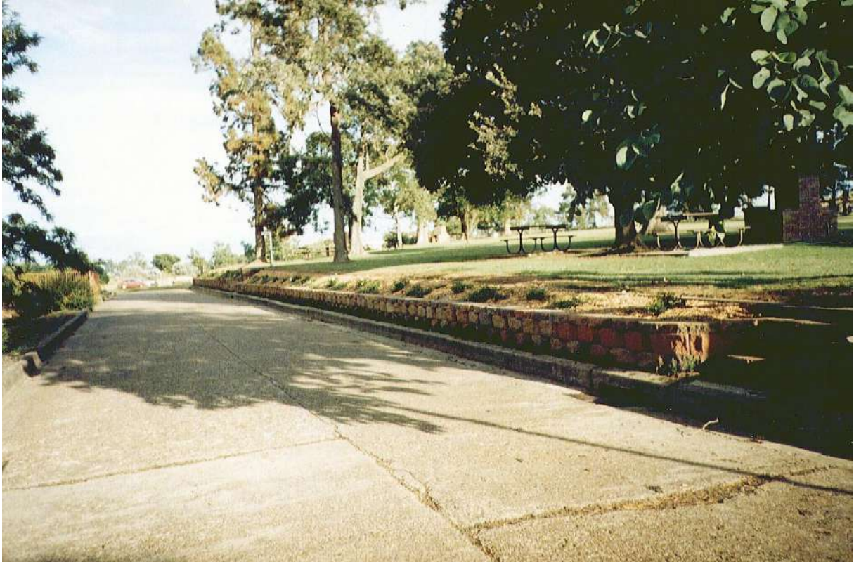
Figure 29: Concrete Block retaining wall built 1999. Photo Provided by MCC
