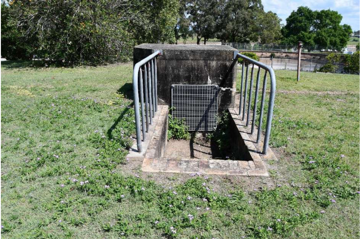
Figure 101: The 1950s pipe access point constructed at the southern end of Filter Bed 4 (Item I-4). The use of brickwork here indicates this may be reusing an early feature as other 1950s period features exclusively use concrete or asbestos. View to the south
