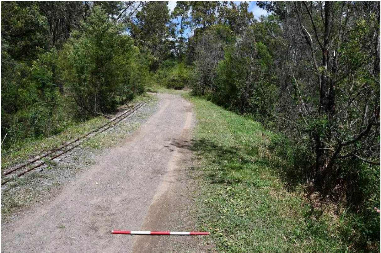
Figure 91: Example of an embankment constructed for the former railway line, now converted to a gravel road and partially utilised by the miniature railway.
