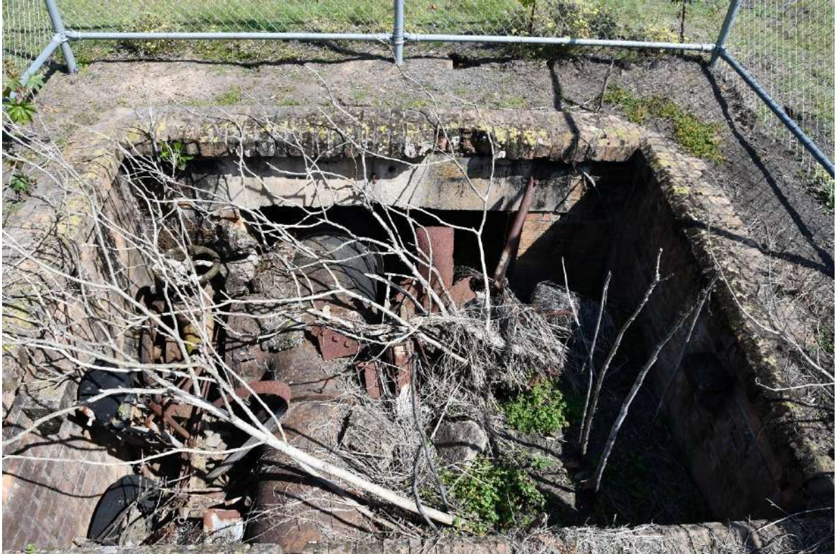
Figure 103: The northernmost exposed section of the central pipe showing it within a sandstock brick lined pit. View to the south
