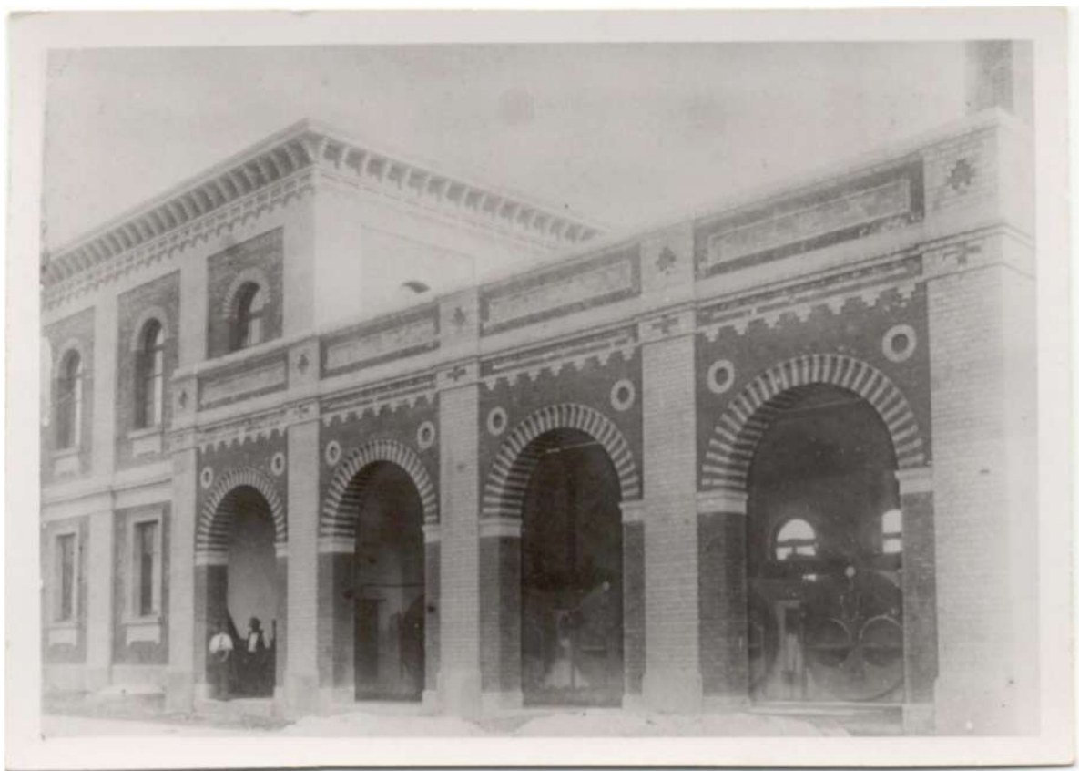
Figure 12: The Boiler Room during operation c.1887-1892 before the construction of the Eastern Annex (1892). Undated photo from the Maitland City Library collection.
