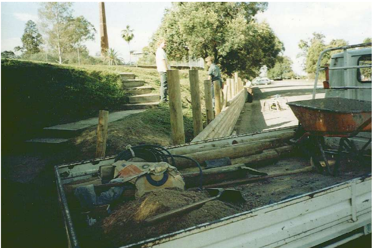
Figure 30: Timber retaining walls built. Photo Provided by MCC
