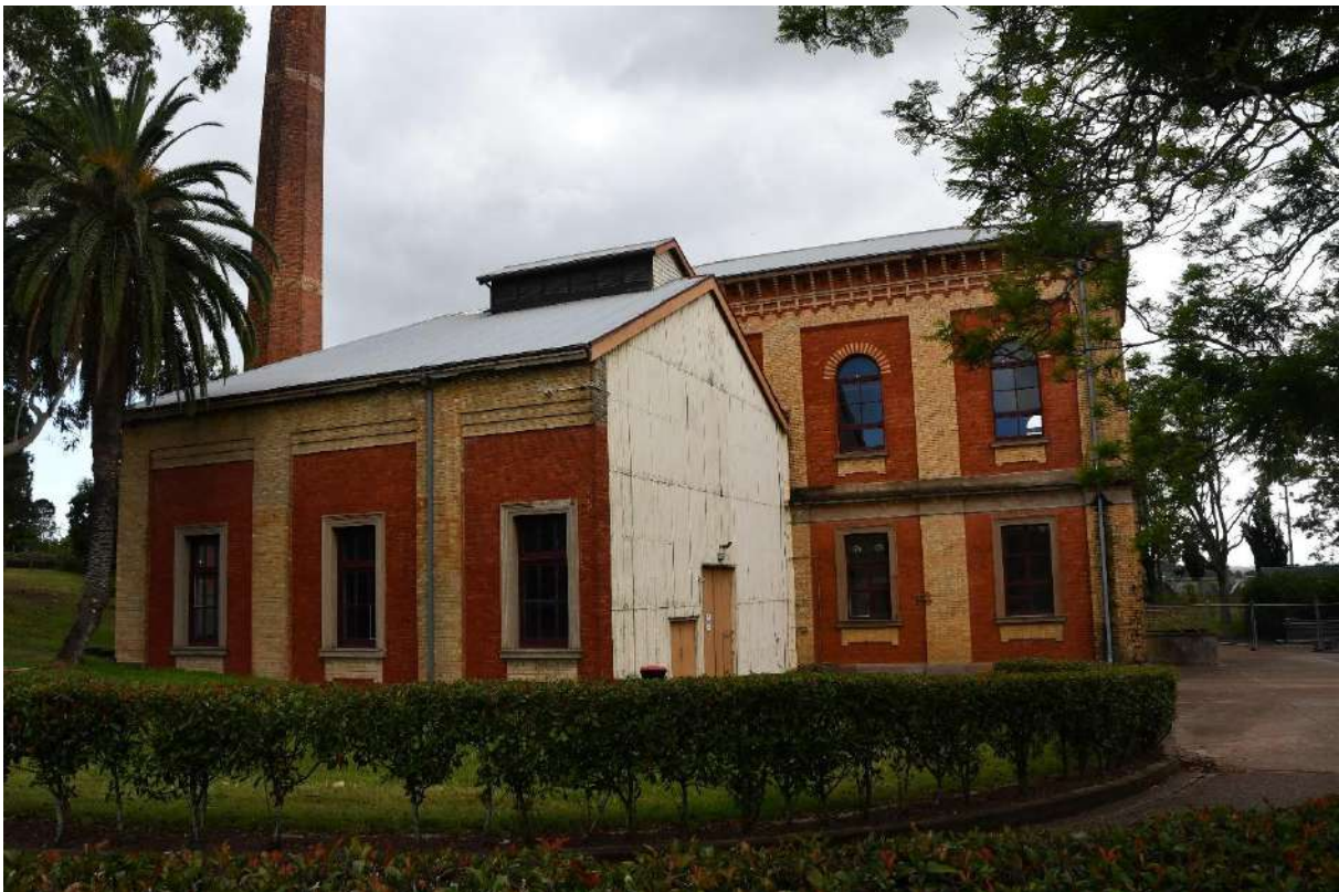
Figure 74: The southern and western elevation of the Pumping Station showing the southern face of the Western Pumphouse (Item F) with its corrugated iron face. View to the northeast
