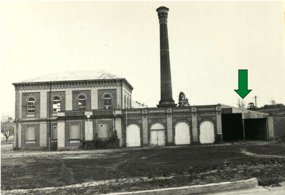
Figure 78: The Eastern Elevation of Pumping Station in 1984. The roof of Item G is still clearly visible between the Boiler Room (Item B) and the Coal Store / Workshop (Item E) at the right of the image (Green arrow). Photo taken from Malnic 1984 p.188
