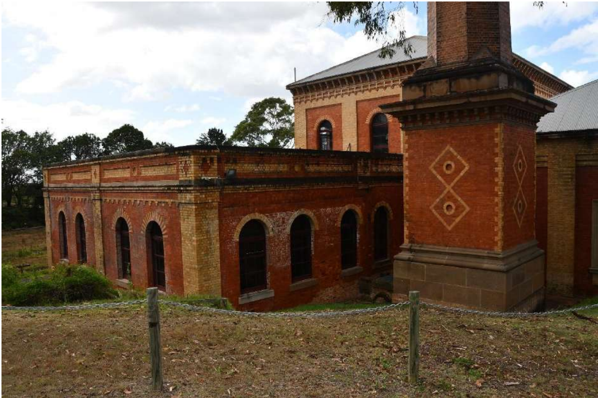
Figure 57: The northern and eastern elevation of the Boiler Room (Item B) showing the paired windows beneath the relieving arches and decorative brickwork.
