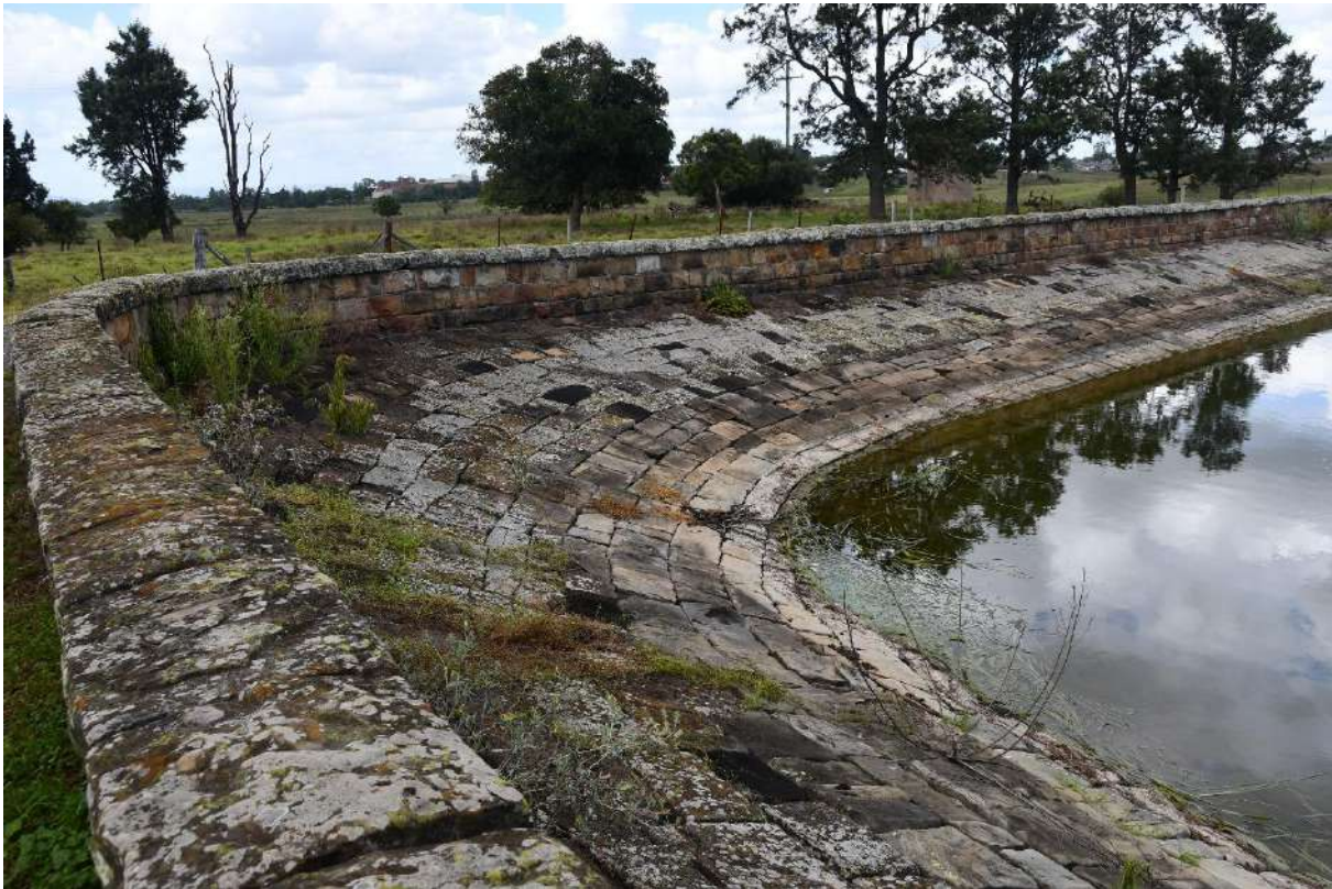
Figure 130: The north facing side of the Embankment showing the well-constructed sandstone elements. View to the southwest.
