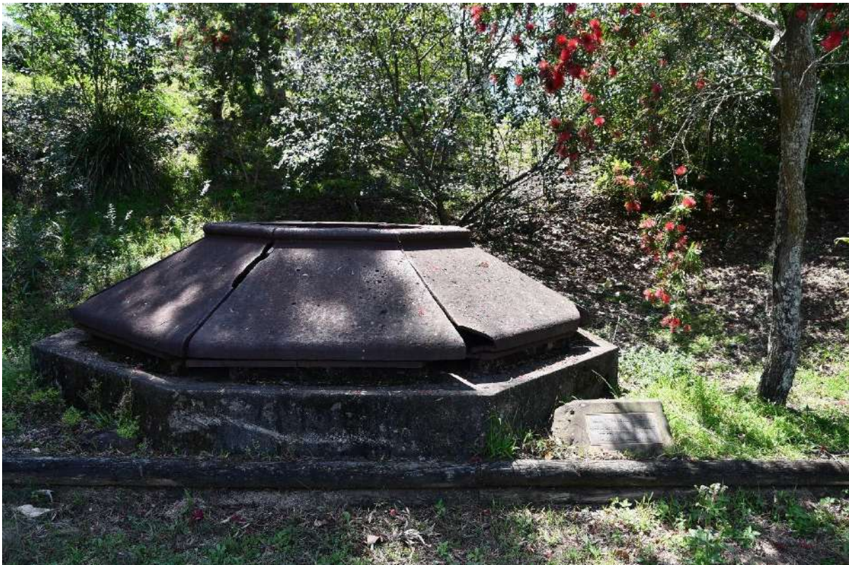
Figure 65: The original cast iron chimney top imported from Scotland, currently located in the Pumphouse Lawn
