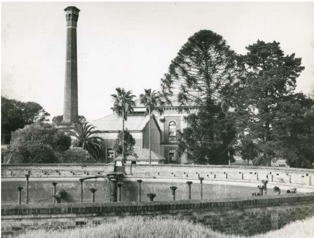
Figure 14: Undated image taken from the Clear Water Tank towards the Main Pumphouse. The roof of the Privy and Change Shed is visible dating the photo to post 1913. Photo from the Maitland City Library collection.
