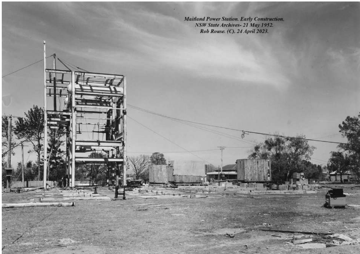
Figure 17: Construction work at the main Power Station site in May 1952. Photo provided by MCC.
