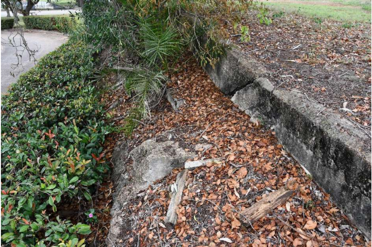
Figure 127: Close up of features along the wall that was likely part of the Sand Washing Plan. View to the north
