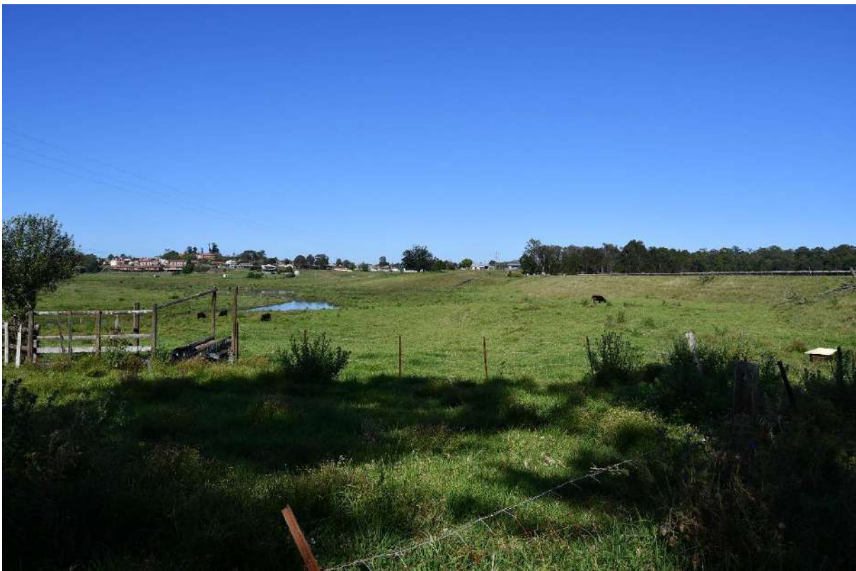
Figure 131: The south facing side of the Embankment which was unlined. The area in the foreground would have been part of the original Walka Logon. View to the west
