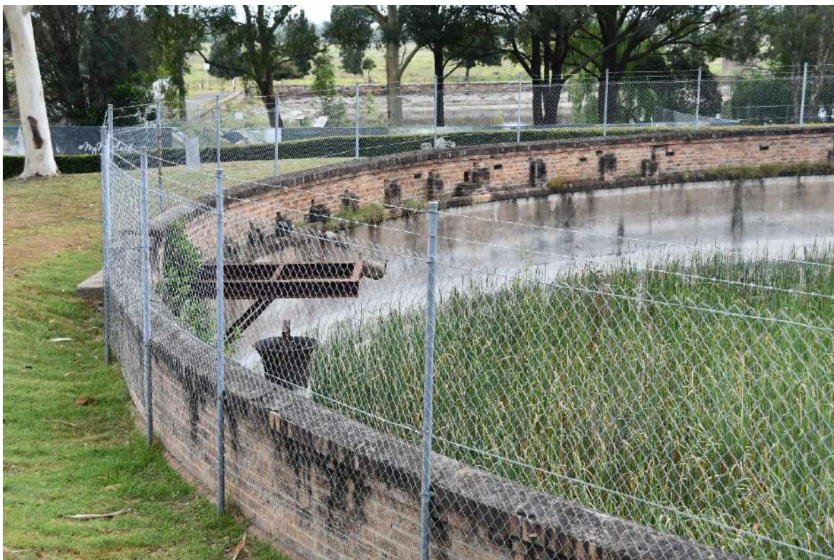
Figure 113: Close up of the inlet and gated entrance to the Clear Water Tank facing south. Some of the internal support pillars are also visible.
