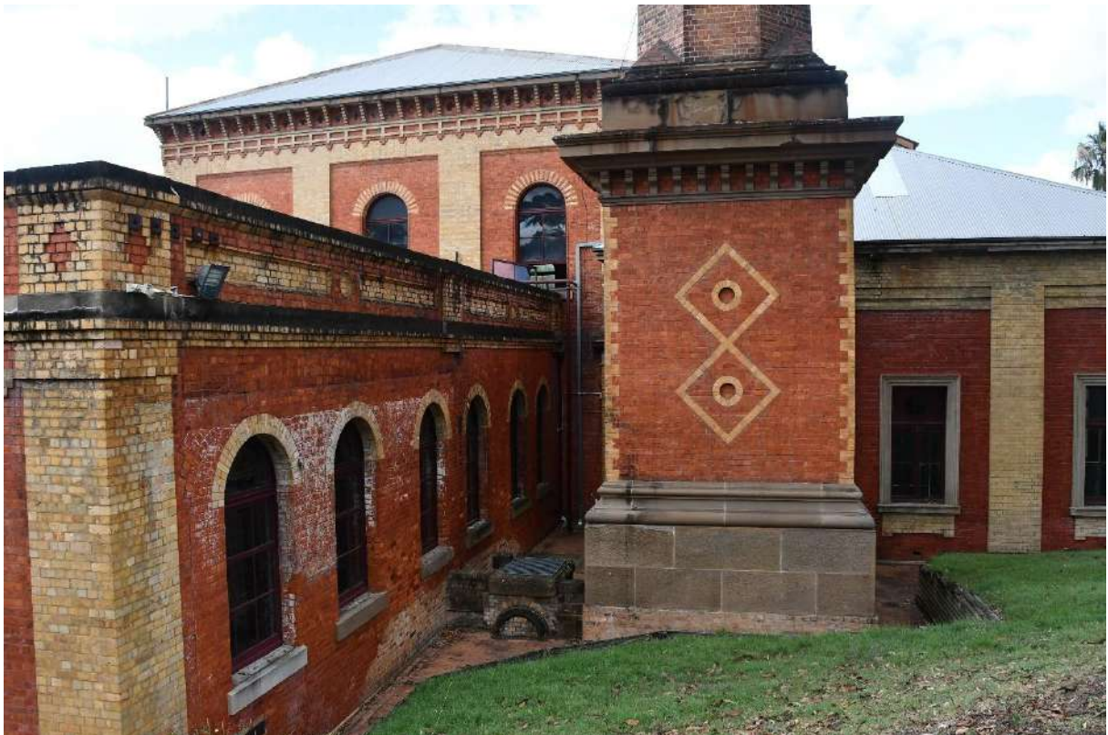
Figure 63: The lower section of the chimney (Item C) viewed from the north with the diamond and circular motif and sandstone base visible.
