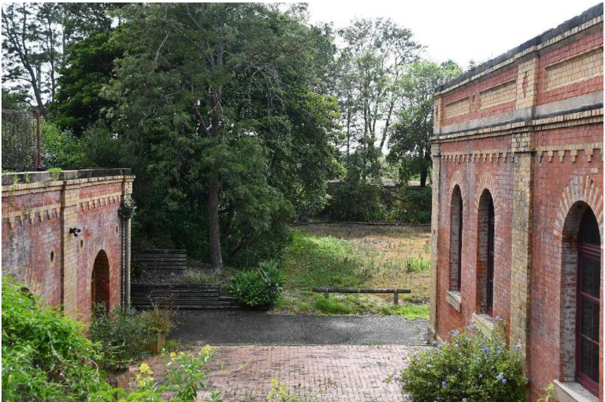
Figure 79: The space between the Coal Store / Workshop (Item E) and Boiler Room (Item B) where the Boiler Room Addition (Item G) was located. View to the east.
