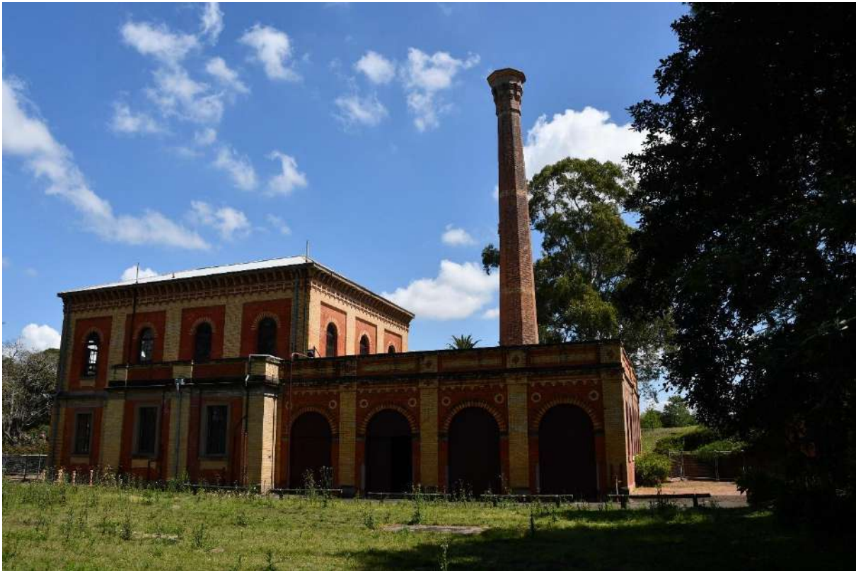
Figure 40: Eastern elevation of the Main Pumphouse (Item A), with Eastern Annex (Item D) and Boiler Room (Item B) visible.
