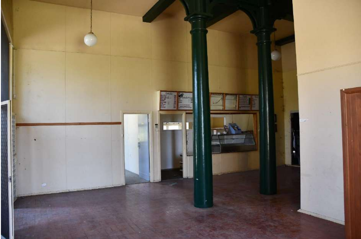
Figure 42: The Main Office (Room #01) in Main Pumphouse (A) looking towards Room #02 and #03. Note the original columns with 1950s floors and internal partitions creating the additional rooms.
