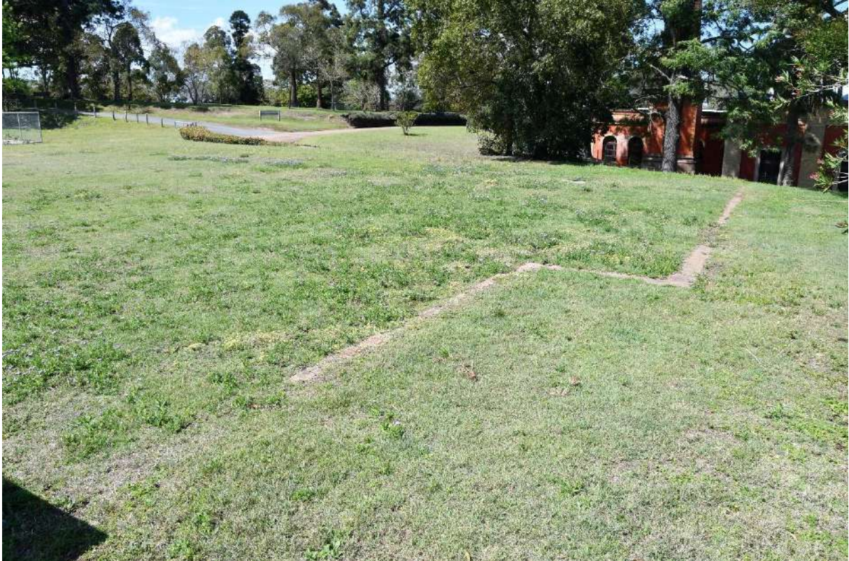
Figure 102: The southeastern corner of Filter Bed 4 (Item I-4) showing the modified footprint caused by the 1950s modifications. View to the east.
