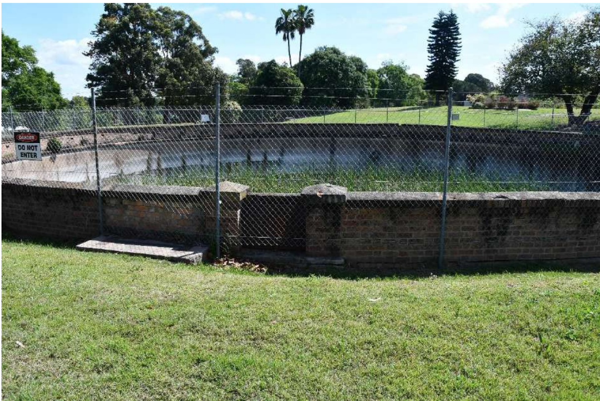
Figure 112: Close up of the gated entrance to the Clear Water Tank on the eastern side. View to the east.
