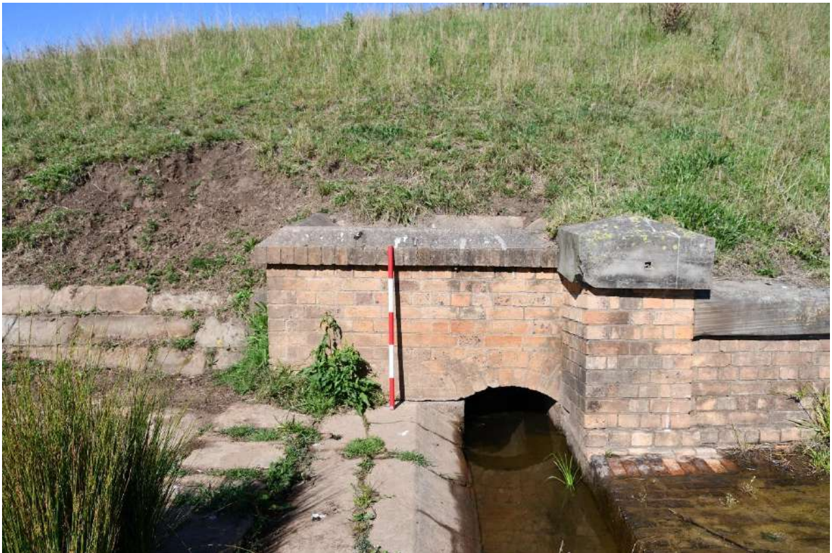
Figure 137: Valve pit at the southern end of the Byewash. View to the west. Scale = 1 metre
