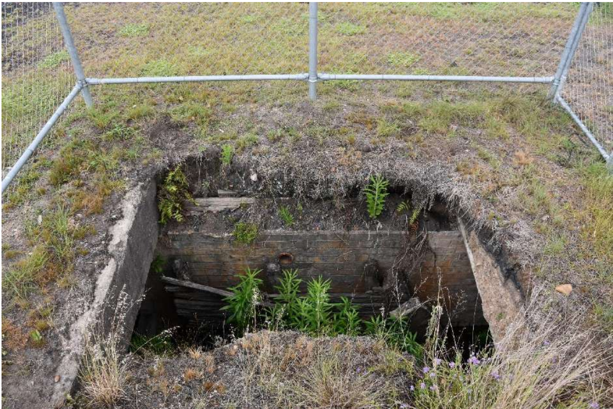
Figure 117: The central access point which is unlikely to be original. The brickwork on the tunnel is clear. The large central iron pipe is obscured by a small collapse of the surrounding topsoil. View to the east
