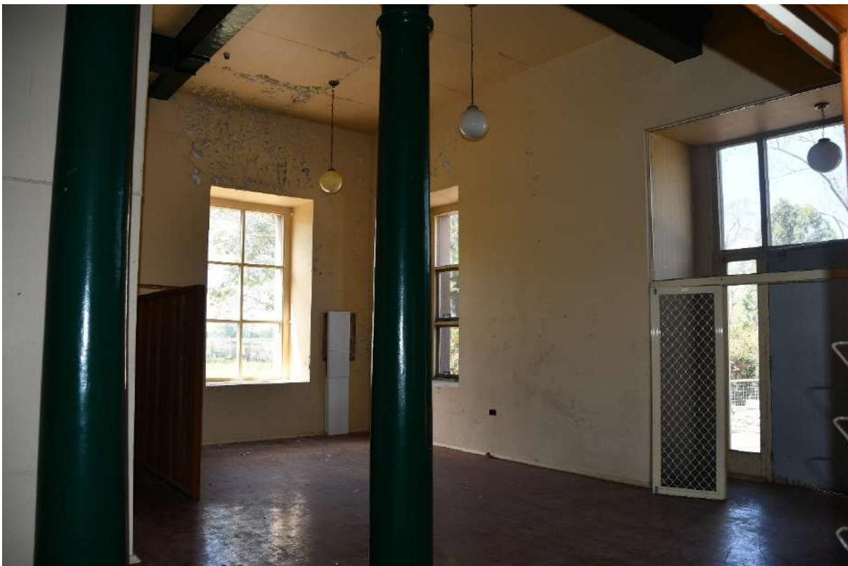
Figure 43: The Main Office (Room #01) looking towards the southeast corner. The entrance into the Main Pumphouse is visible. There is some paint flaking around the windows along with mould but otherwise, the room is in good condition.
