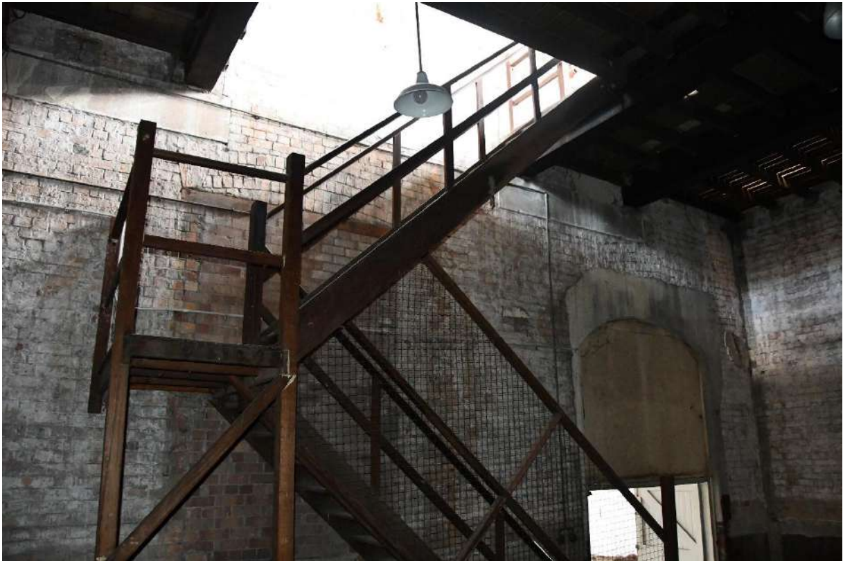
Figure 48: The 1950s internal staircase that links Room #04 to Room #09 above.
