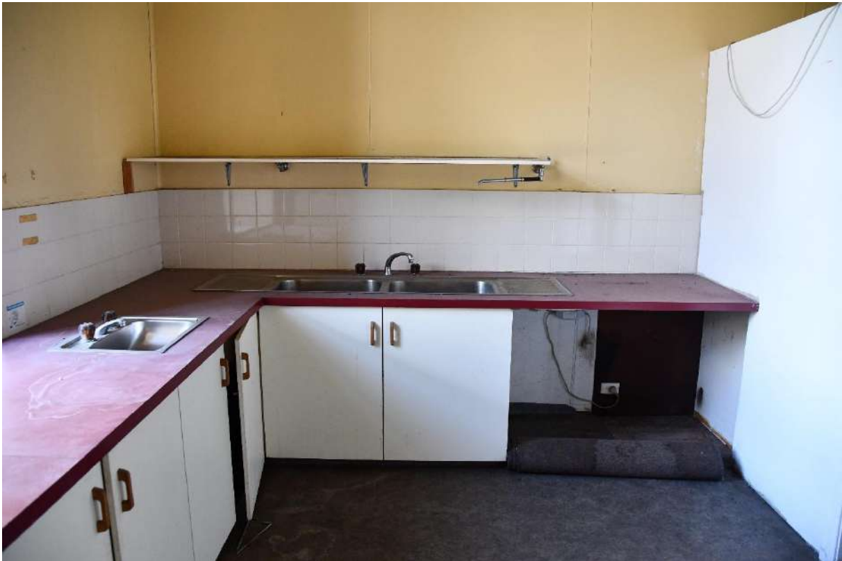
Figure 46: The rear area of Room #03 showing the 1990s cabinetry and sinks.
