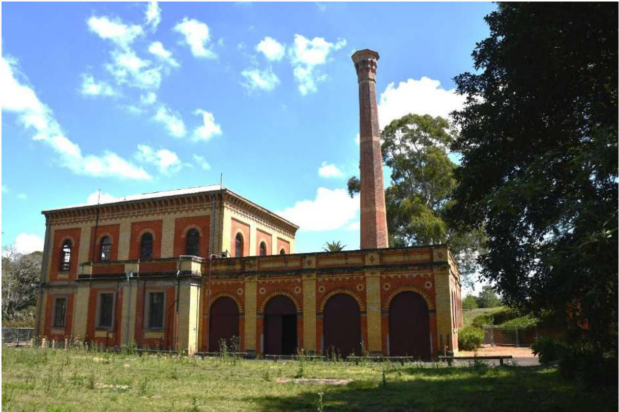
Figure 55: The eastern elevation of the Main Pumphouse (Item A), Eastern Annex (Item D) and Boiler Room (Item B). The four pilastered arched doorways with modern doors are visible. View to the west
