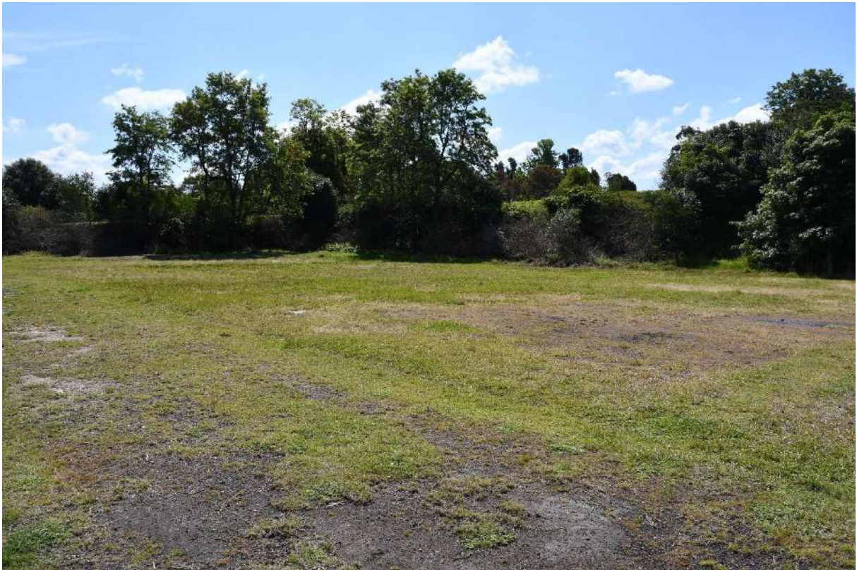
Figure 108: Filter Bed 7 (item K-7), as viewed from the southeast. This Bed is largely only visible as a rectangular parch mark.
