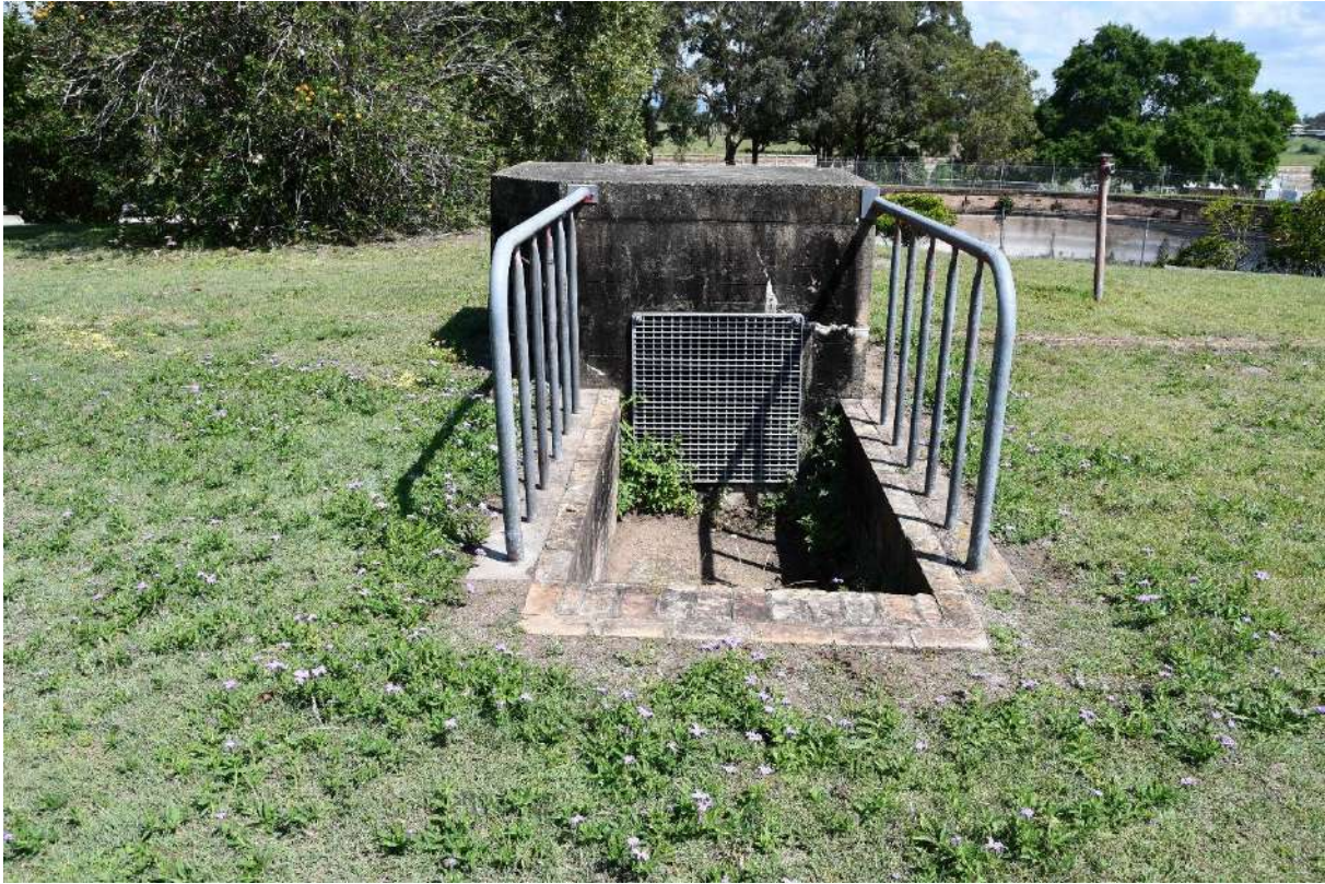
Figure 120: The c.1950s above ground pipe access point. This was likely part of the cooling system for the Power Station. View to the south
