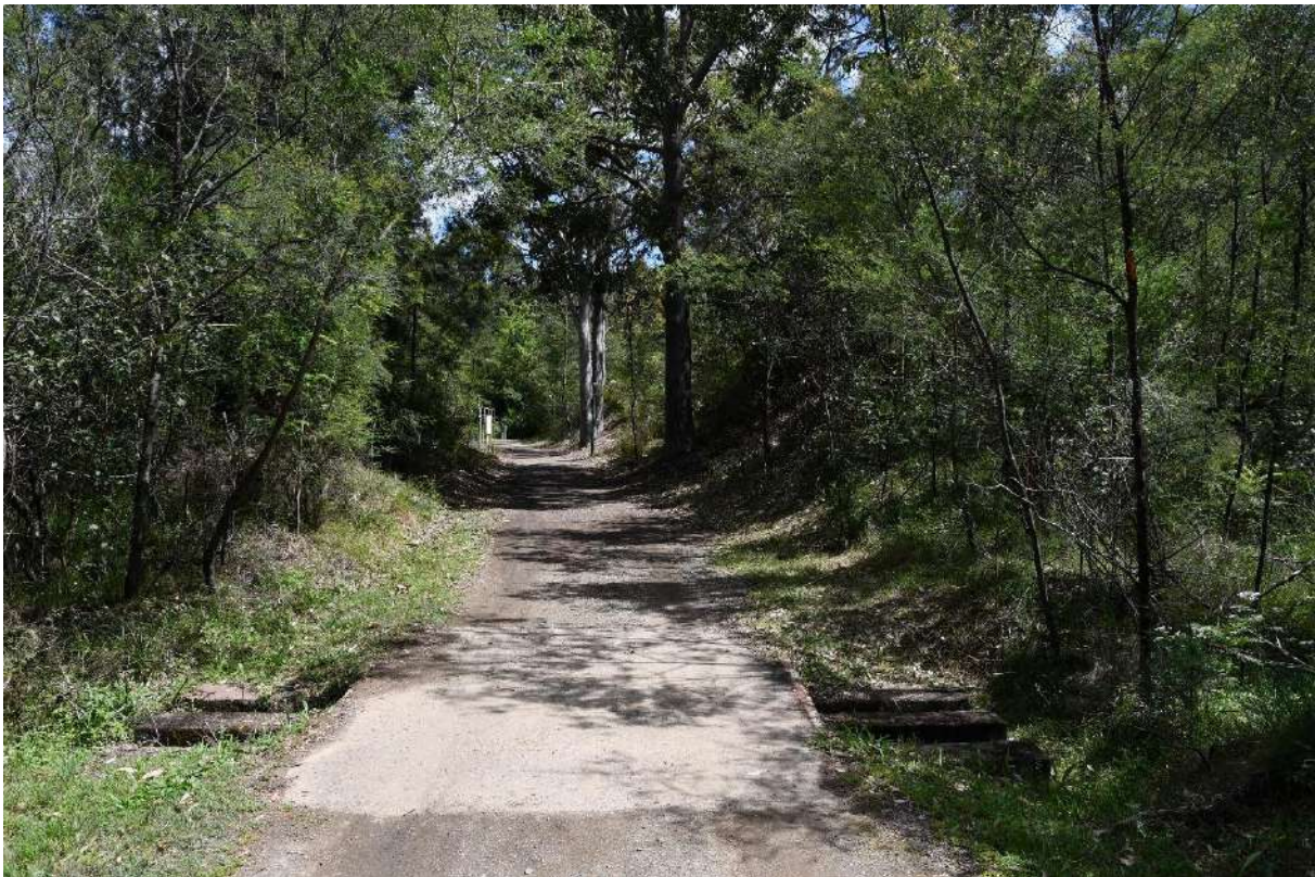
Figure 93: View along the former railway showing the small nature of the bridges.
