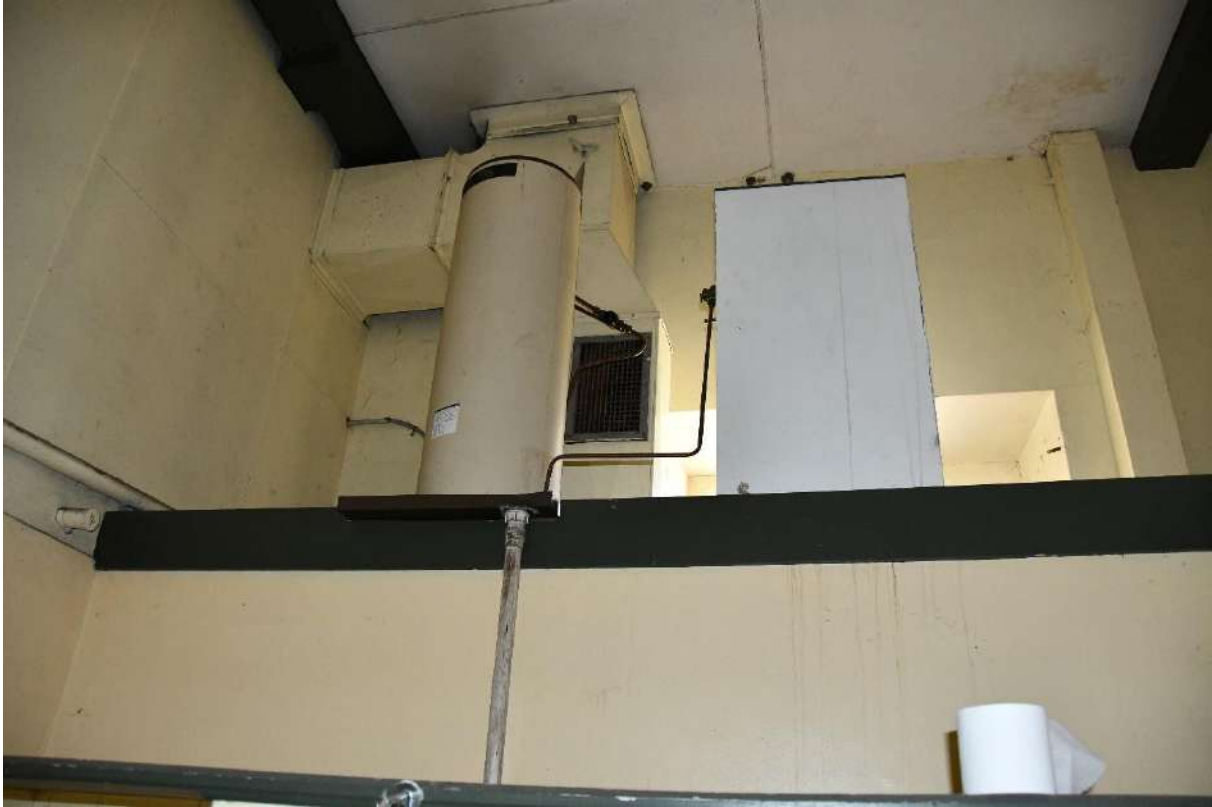
Figure 50: The false ceiling and various vents within the Toilets (Room #05)
