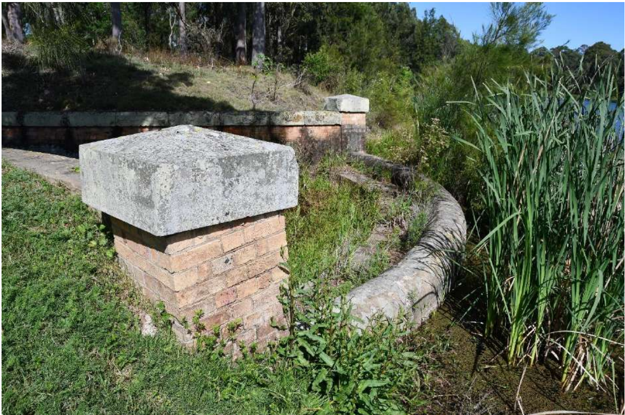
Figure 135: The curved opening of the Byewash within the Reservoir with the well-constructed sandstock pillars and walls visible, along with the well-formed stonework. View to the west.
