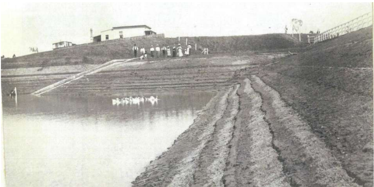
Figure 15: Showing the aftermath of the flood of 1893. The Second Engineers residence is visible on the high ground. Photo provided by MCC.
