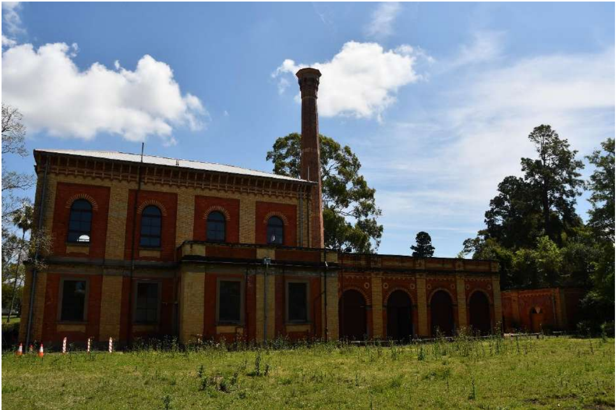
Figure 20: Eastern face of the main building showing the Main Pumphouse (A), Eastern Annexe (D) and Boiler Room (B)
