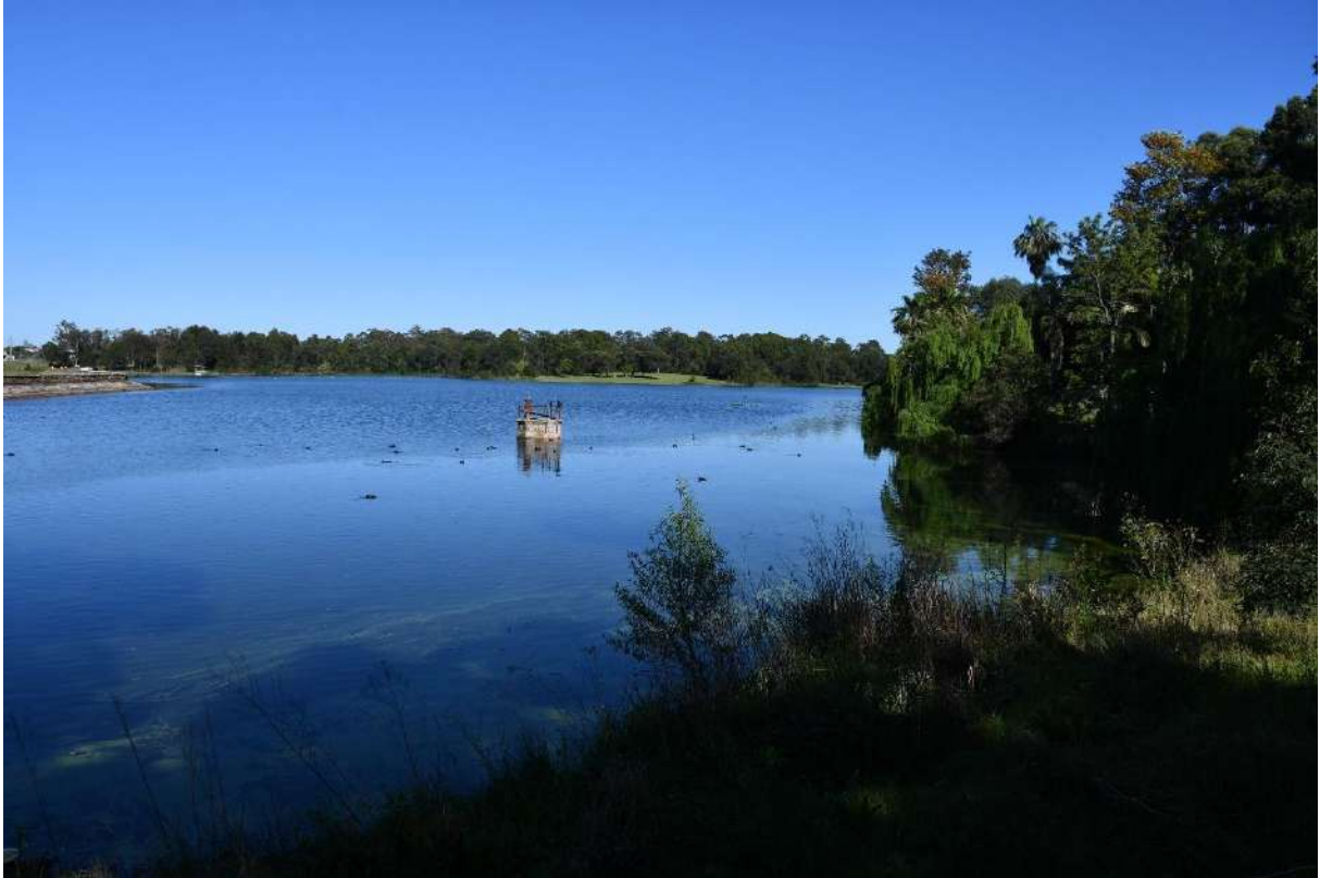
Figure 39: Outlet tower (M)
