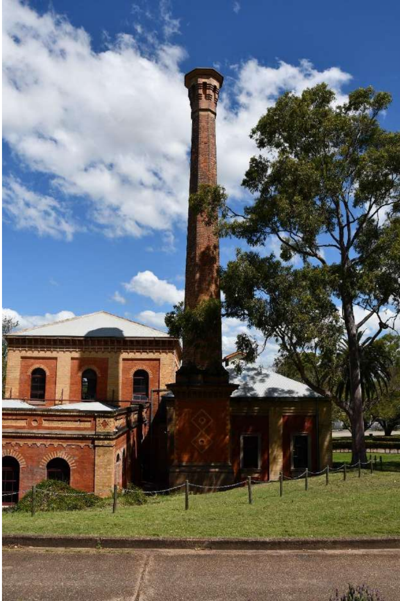
Figure 22: The Chimney (C)
