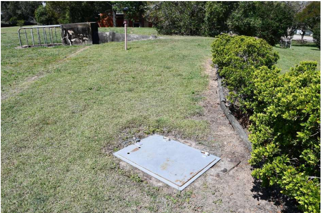
Figure 40: Examples of the Pipe Access Pits (N)
