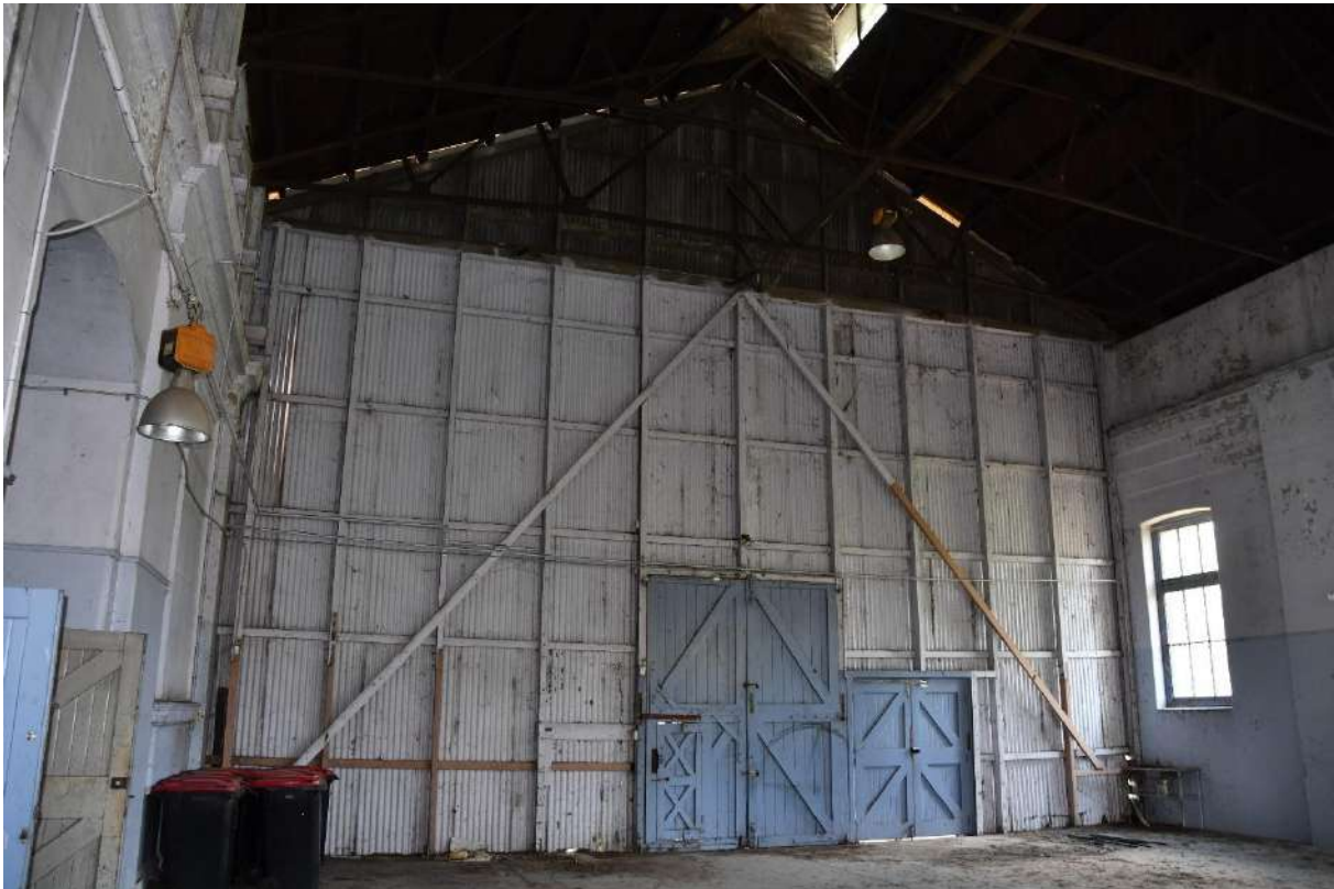
Figure 27: Internal space within the Western Pumphouse (F)
