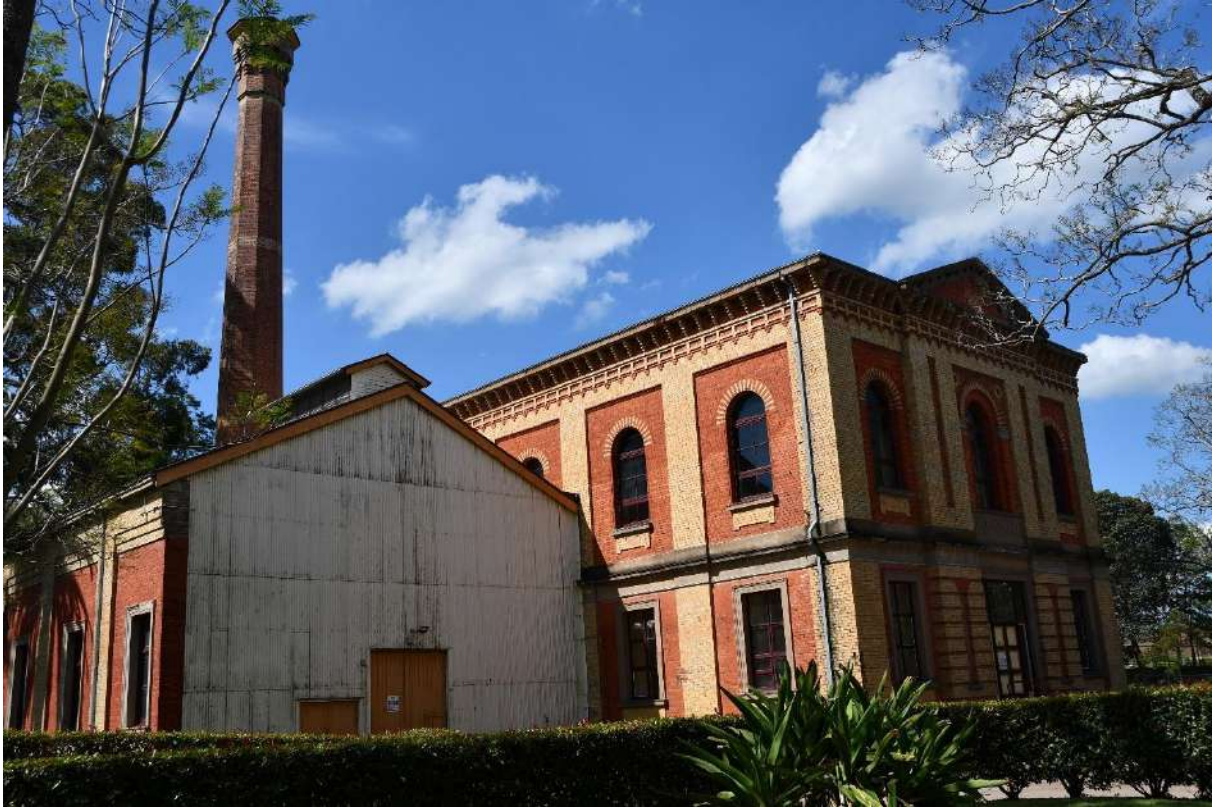
Figure 16: Main Pumphouse (A) and Western Pumphouse (F)
