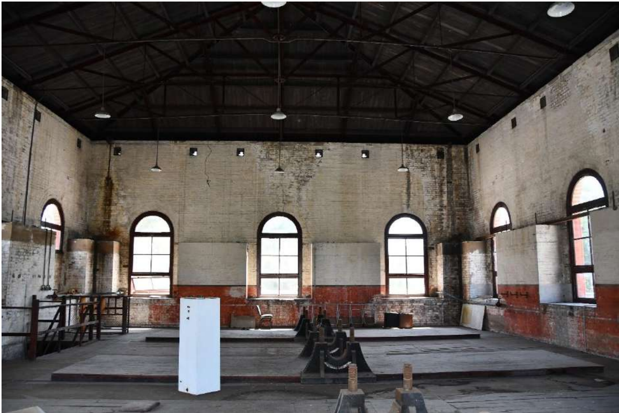
Figure 18: First Floor of Main Pumphouse with original floors and bearing blocks (A)
