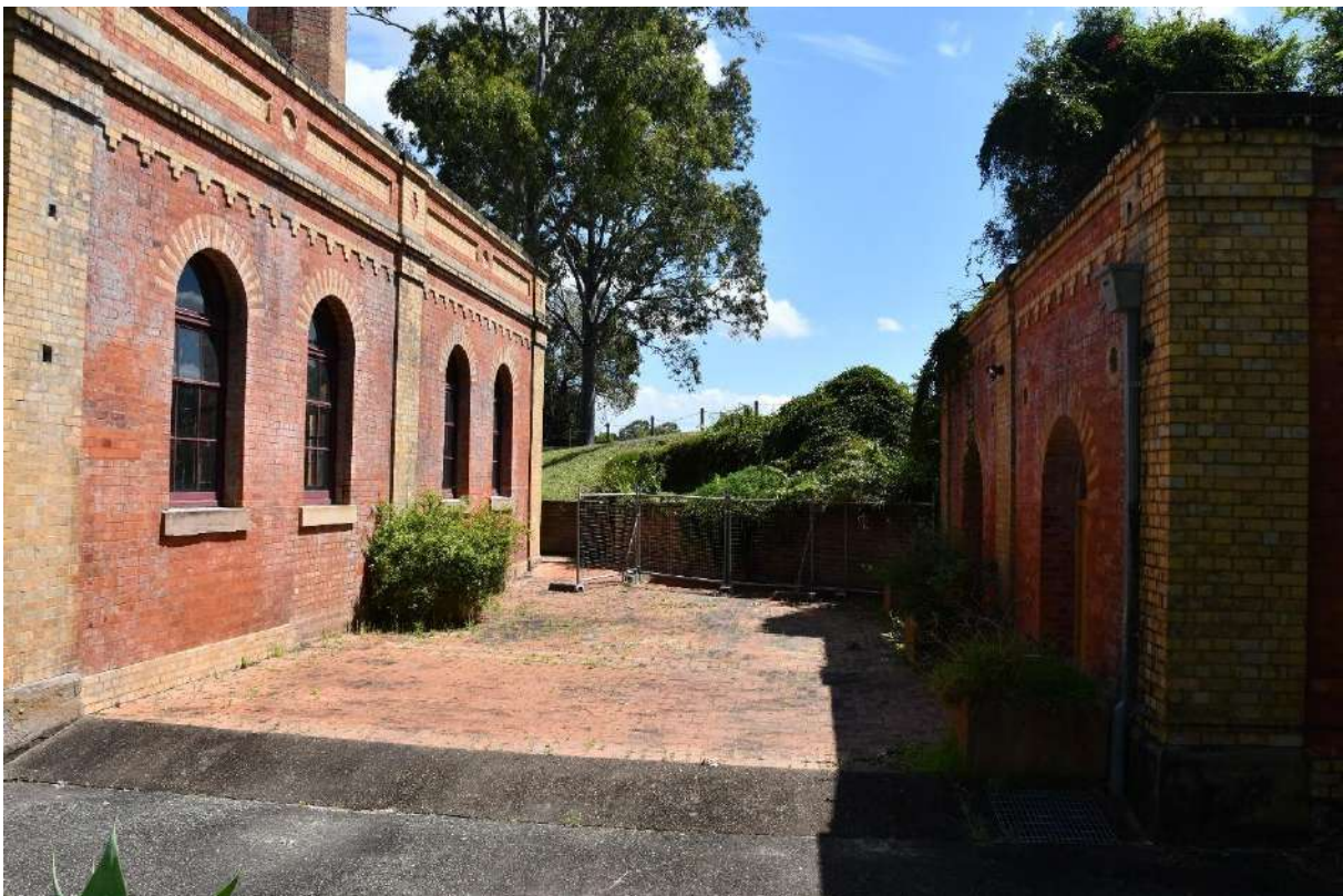
Figure 28: Space where the Boiler Room Addition (G) was located. Note the voids in the northern wall of the Boiler Room that would have supported the roof. The embankment in the background is the location of Pumphouse Number 6 (R)
