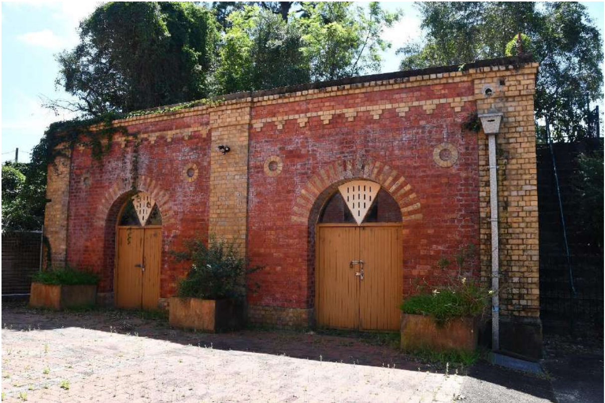
Figure 25: The Workshop / Coal store (E)
