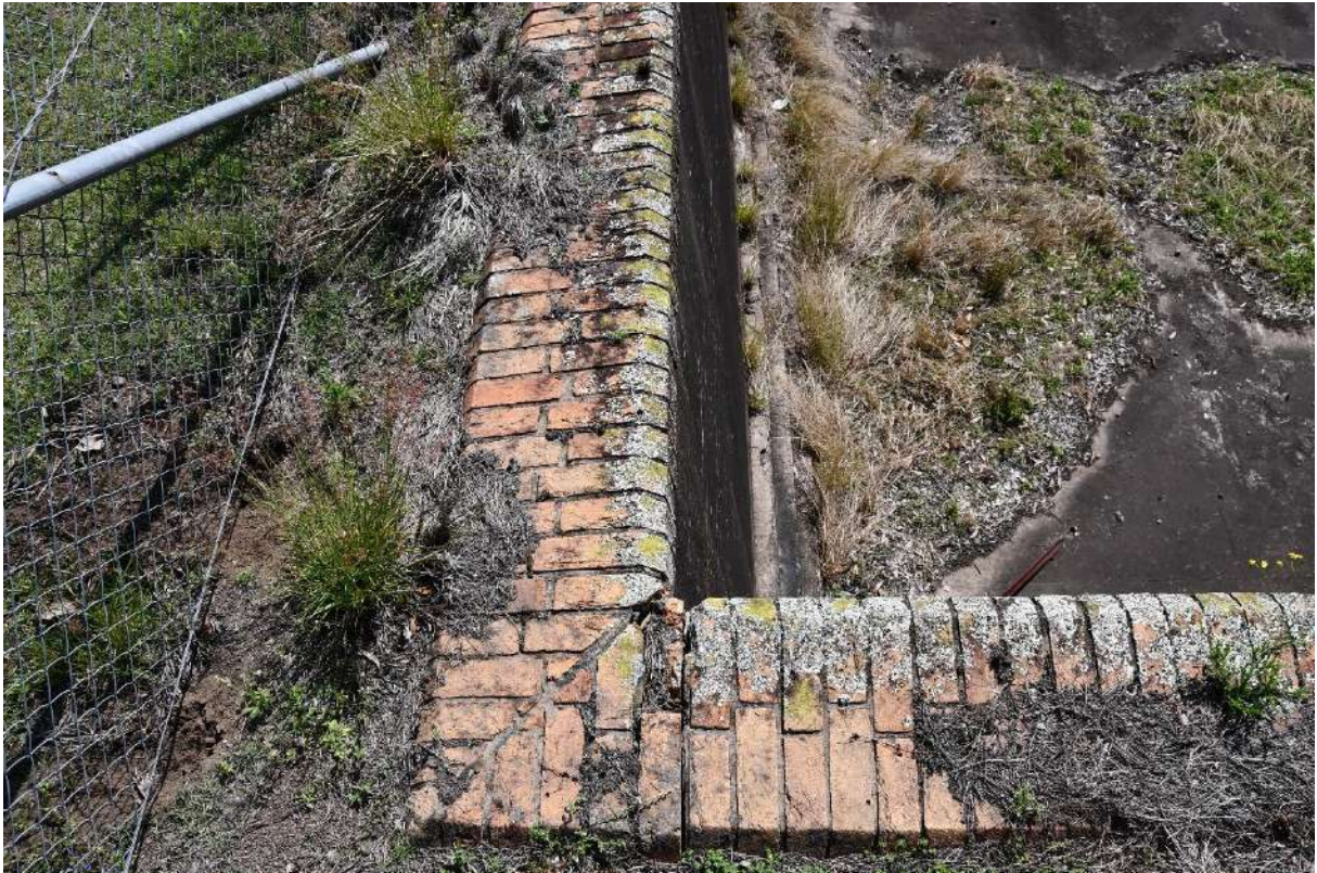
Figure 30: Close up of the brick work in the settling tank (H)
