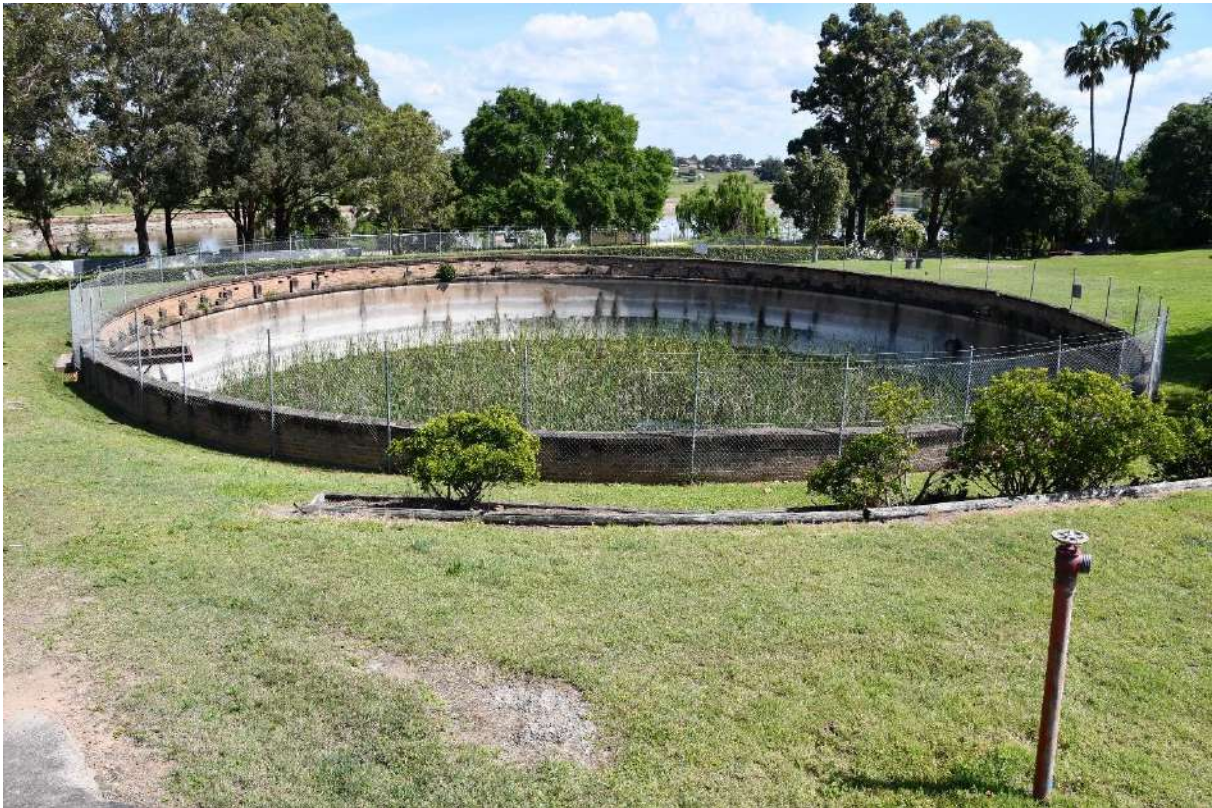
Figure 37: Clear Water Tank (L)
