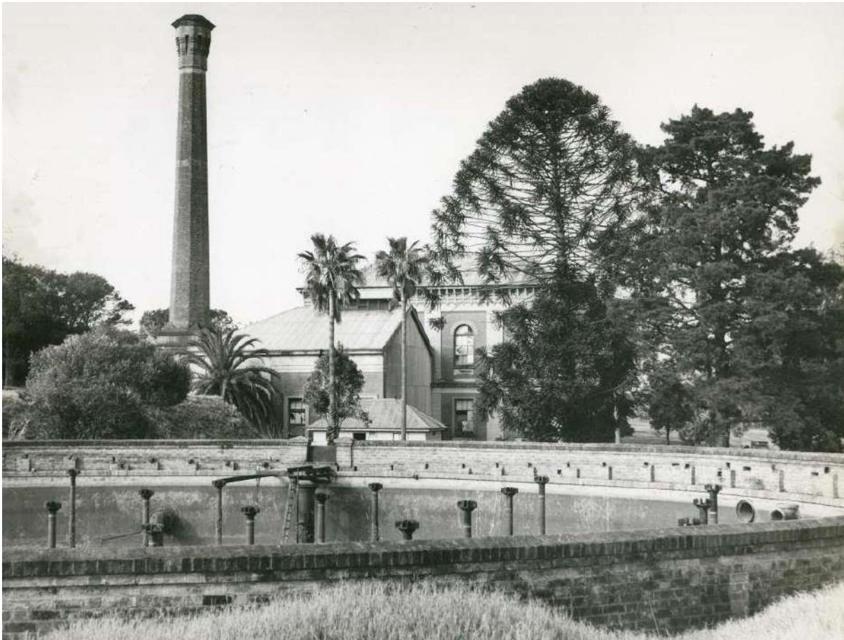
Figure 13: 1947 image of the Cler Water Tank showing the internal roof supports. The roof of the Change Sheds is visible in the background. Photo supplied by MCC
