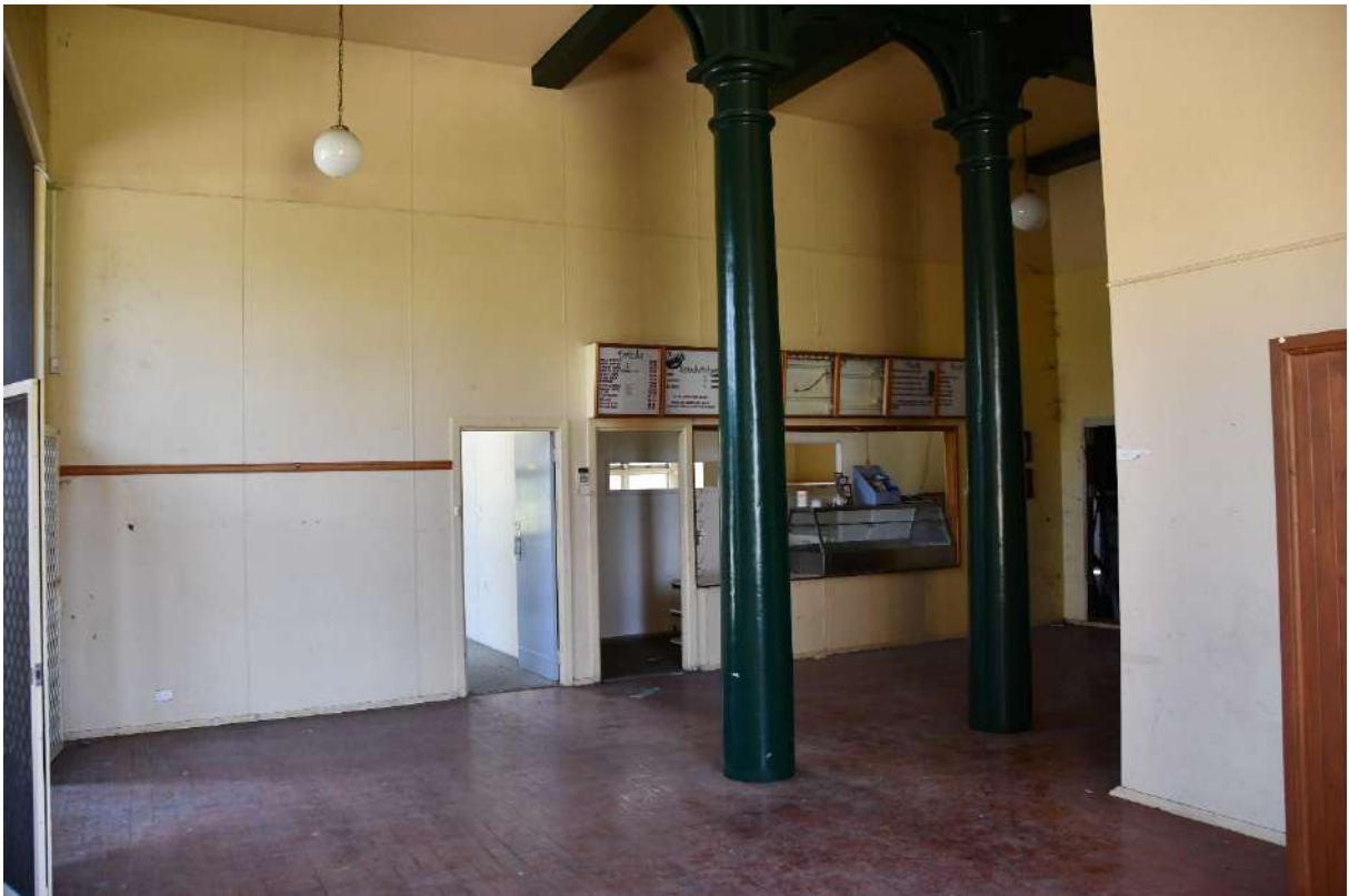
Figure 17: Internal space in Main Pumphouse (A). Note the original columns with 1950s floors and internal divisions in conversion to offices.
