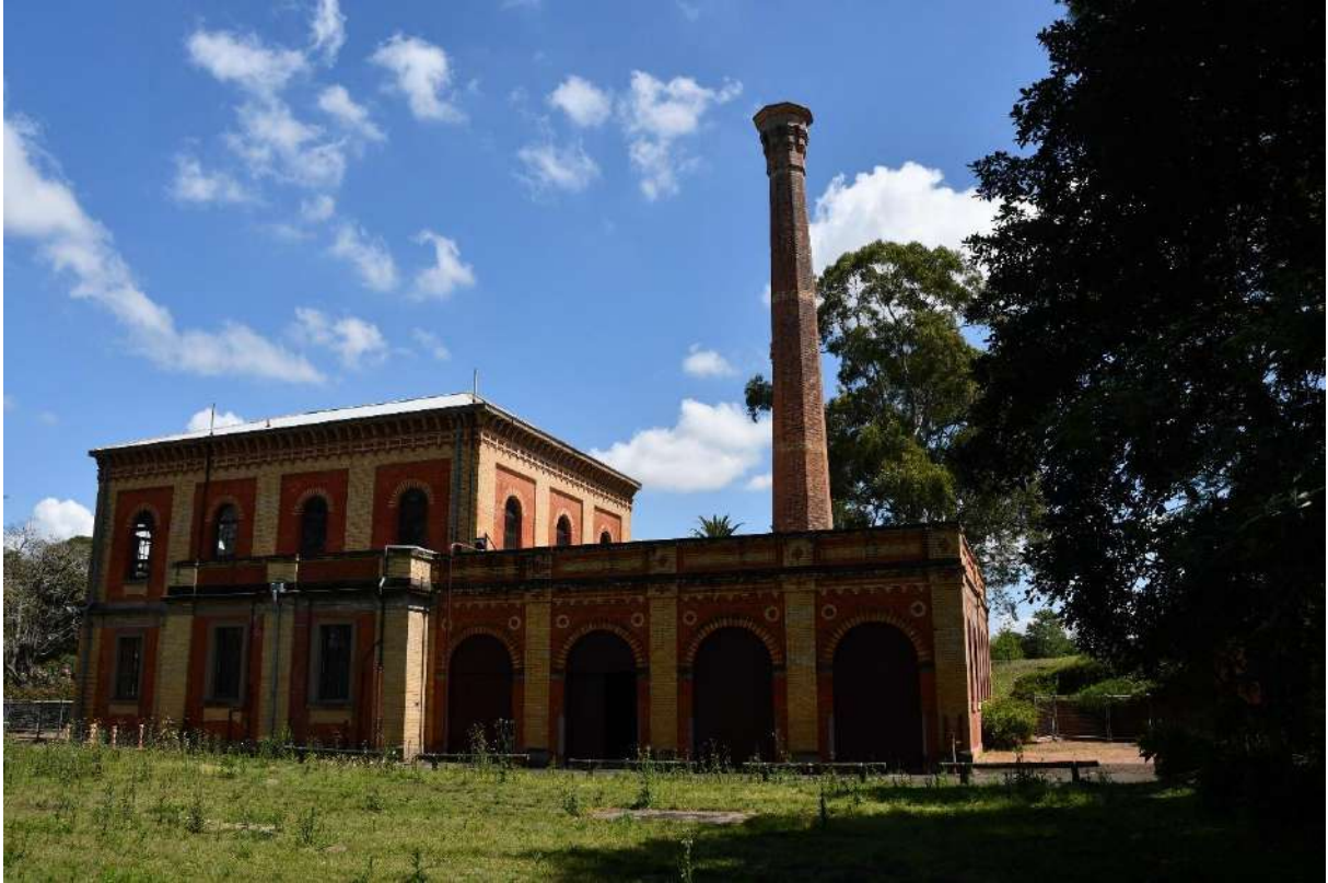
Figure 23: Eastern face showing Boiler Room (B) and Eastern Annex (D)
