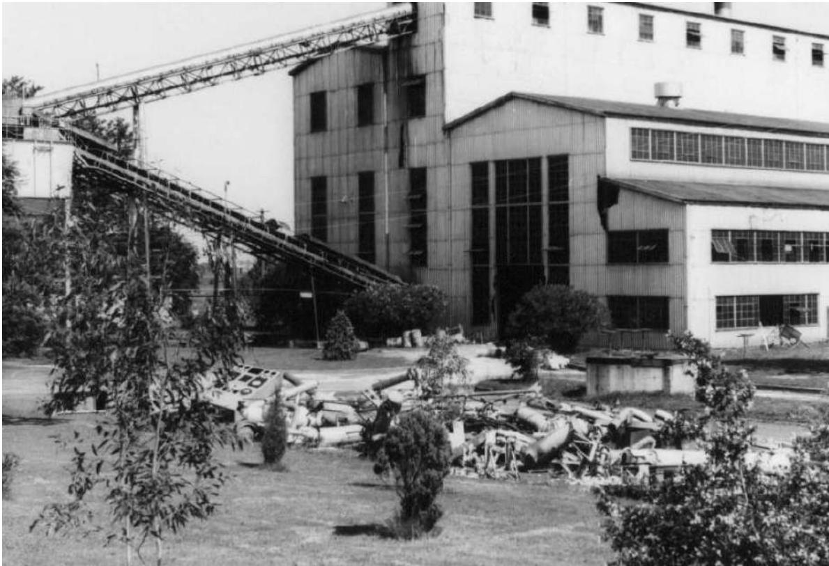
Figure 15: Power Station at the commencement of demolition in January 1978. Image taken from Corkery Consulting 2009
