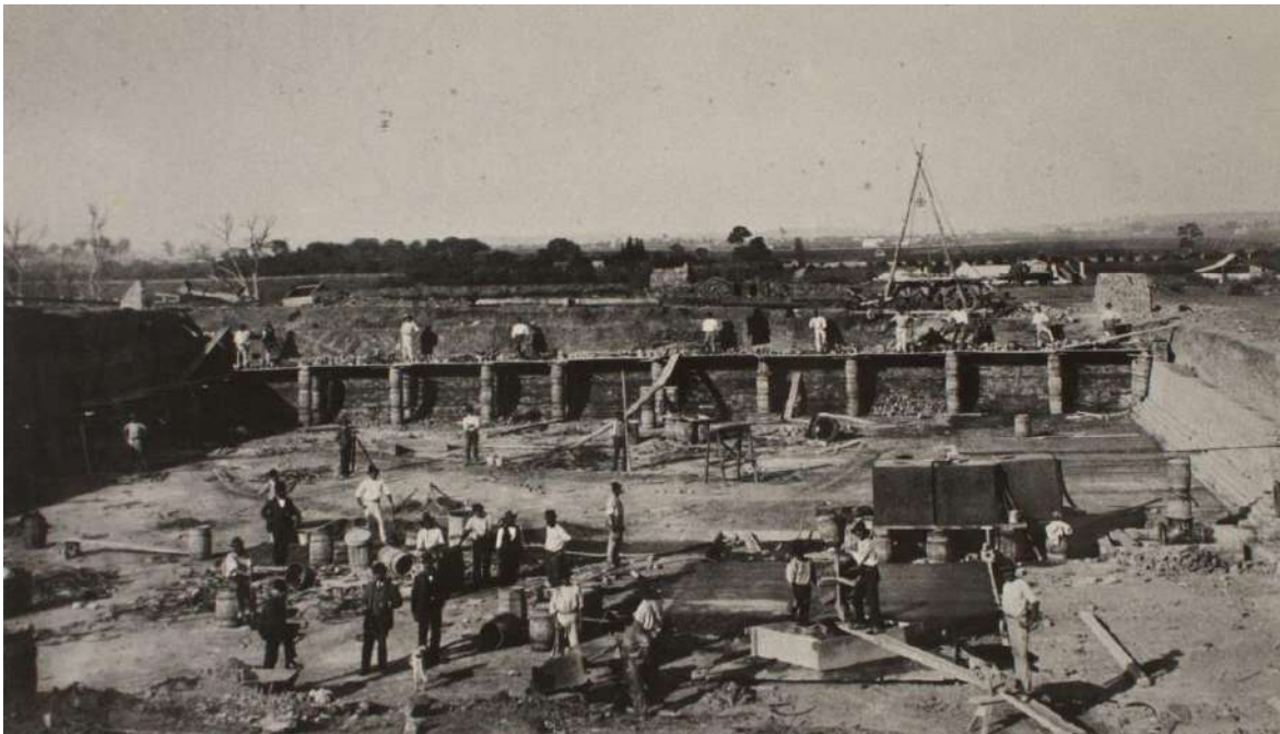
Figure 11: Construction of the setting tank in 1885. Showing the construction methods and materials employed. Photo supplied by Maitland City Council
