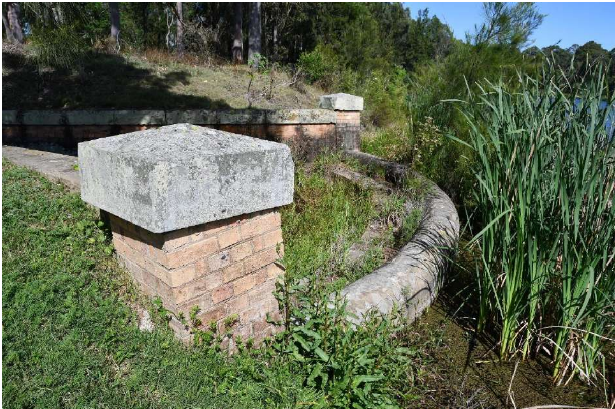
Figure 52: Inlet of the Byewash at the Reservoir (X)
