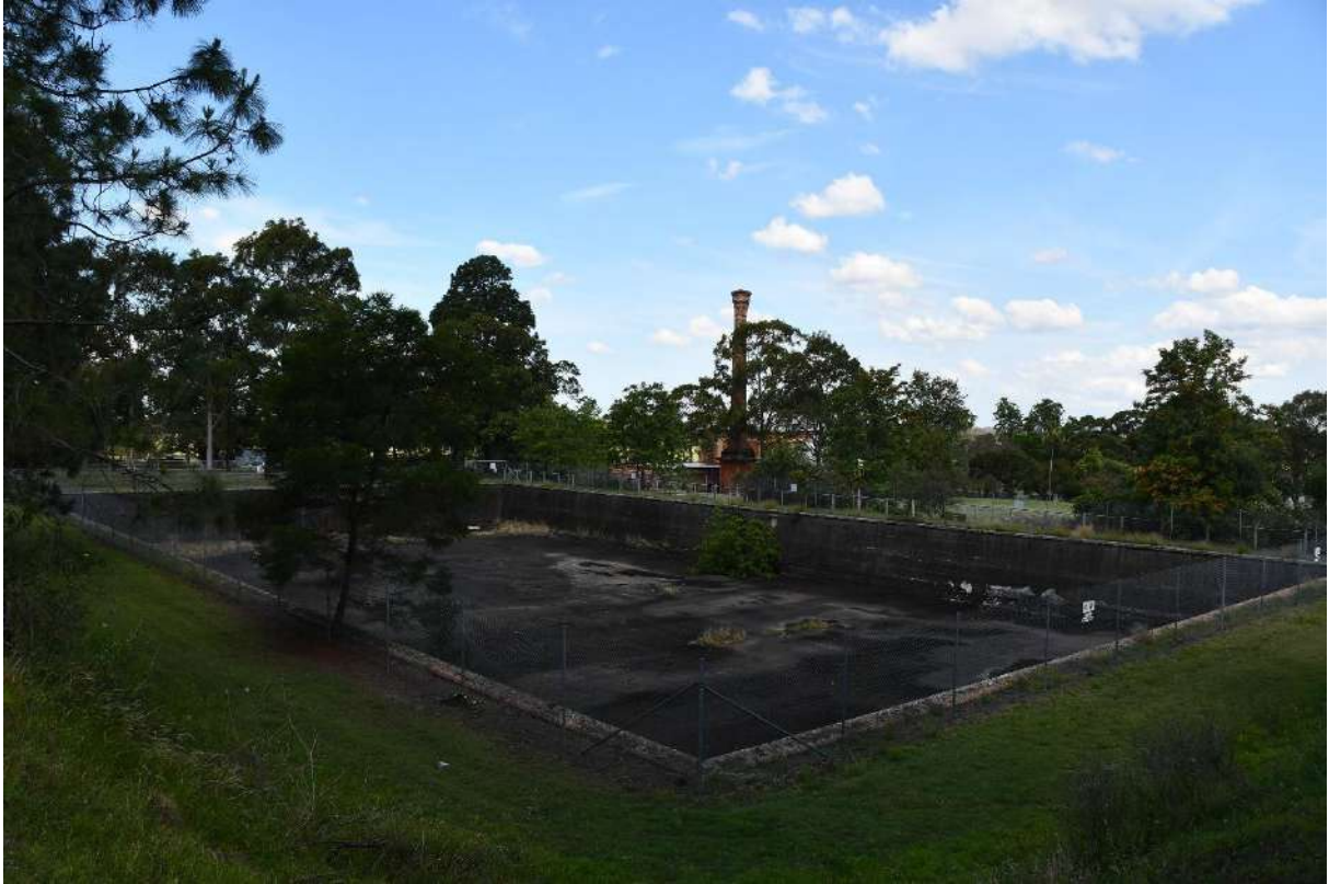
Figure 29: The Settling Tank (H)
