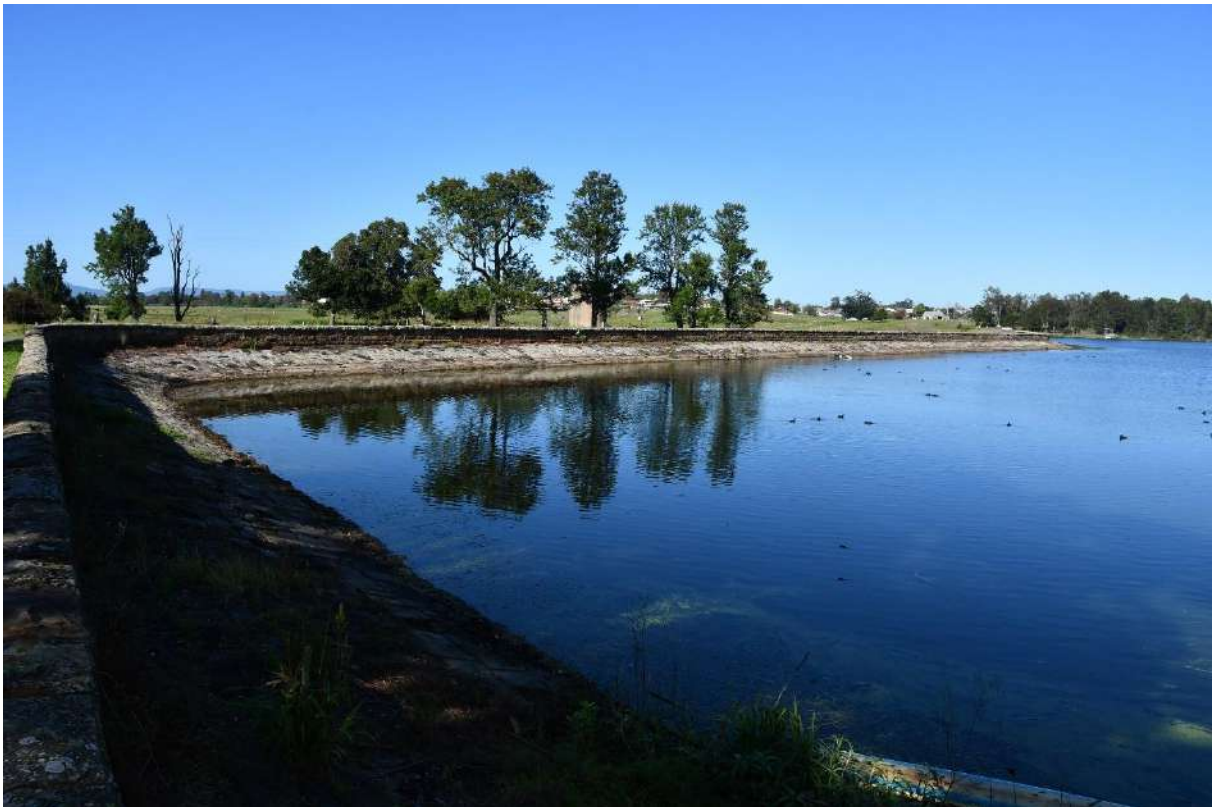
Figure 38: Reservoir Wall (M)
