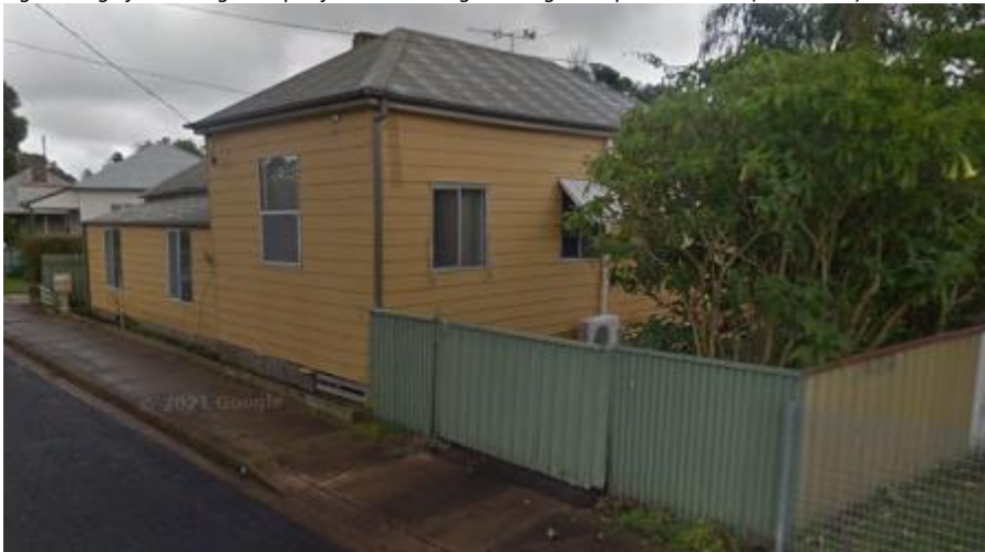
Fig.10 – Image from Google Maps of house existing at 9 Raglan St prior to demo (June 2015).
