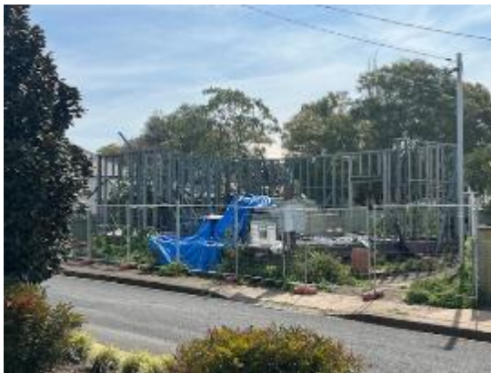
Fig. 3 - View from carpark in Raglan St to the site.
