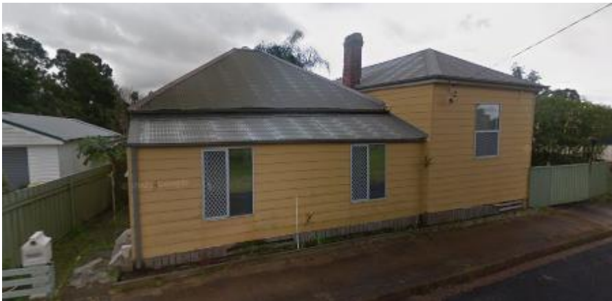
Fig.9- Image from Google Maps of house existing at 9 Raglan St prior to demo (June 2015).
