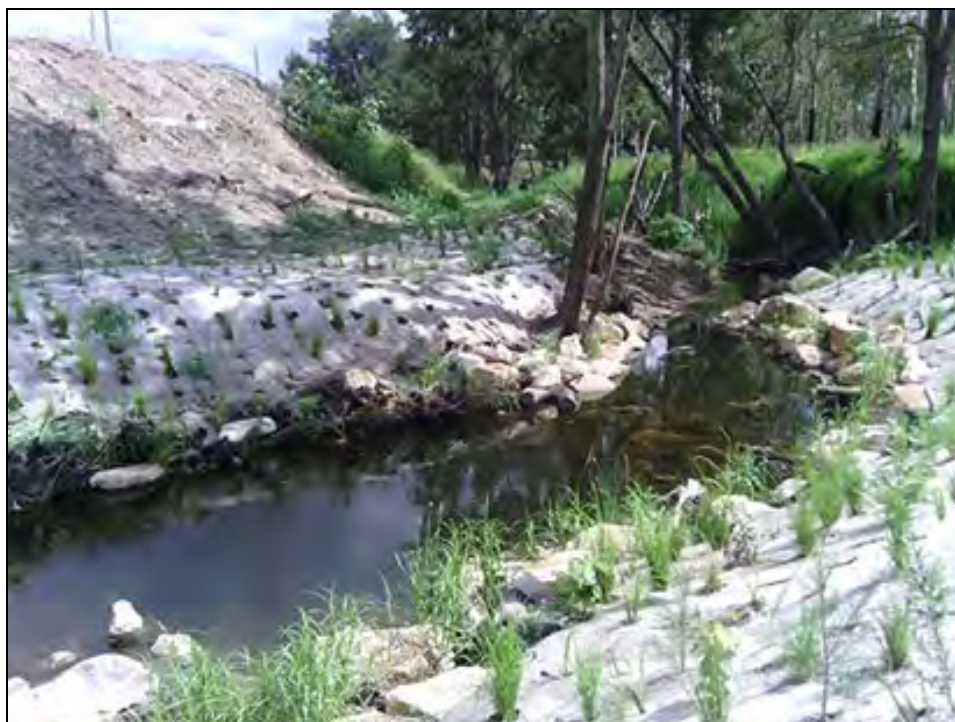
Plate 2 – Bundamba Creek Regeneration works (Australian Wetland Consulting, 2018)
