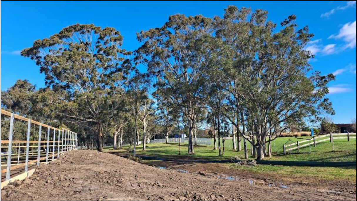
Plate 4 Above: Site photo showing change in ground levels and conditions.
