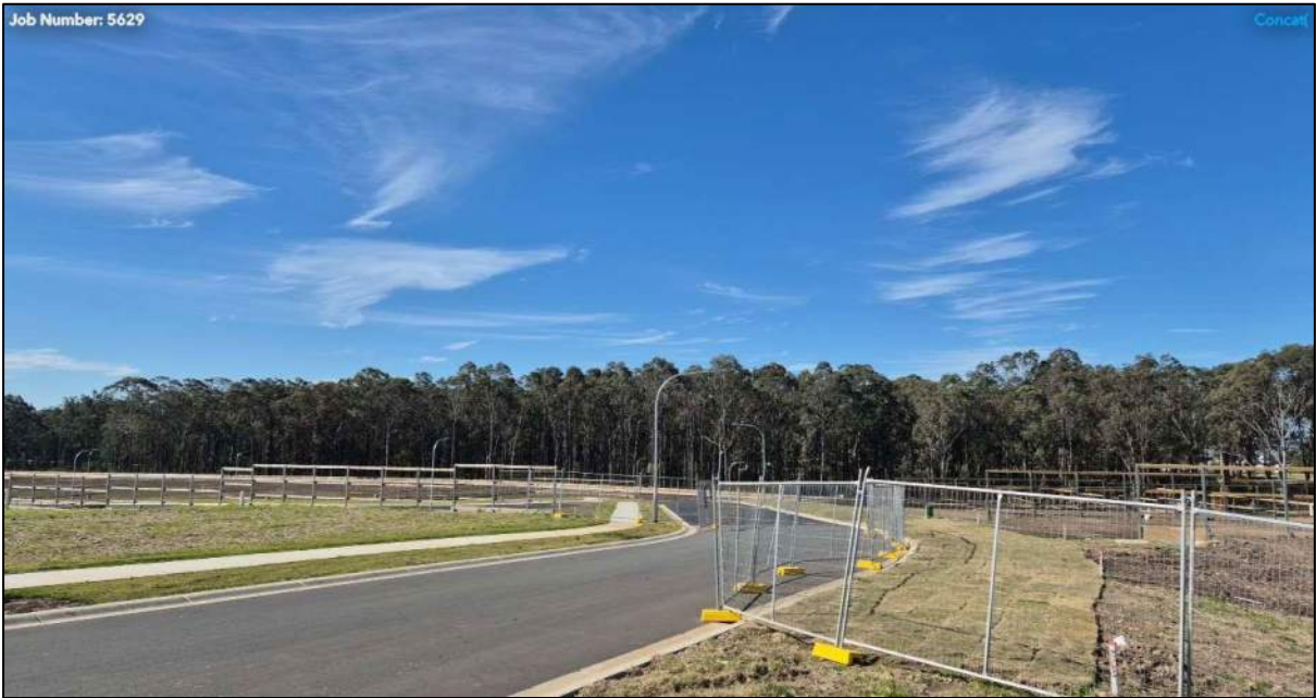
Above: Photo Point 7 - Extension of Cora Way into previously completed stage of the larger residential subdivision.
