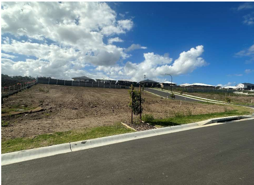
Construction of Multi Dwelling
