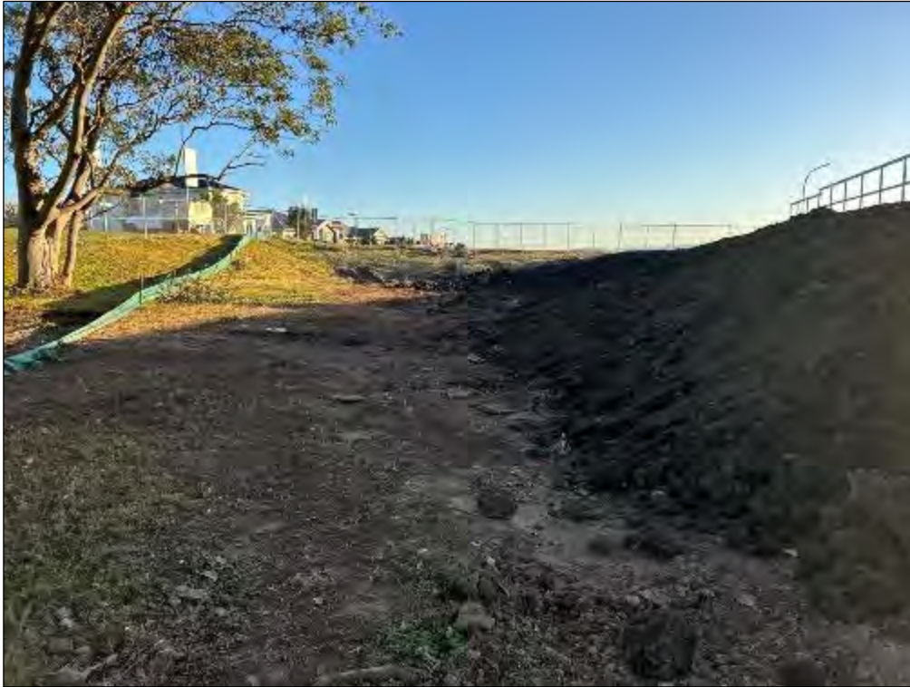
Above: Infrastructure and clearing along the north-east boundary of the Study Area
