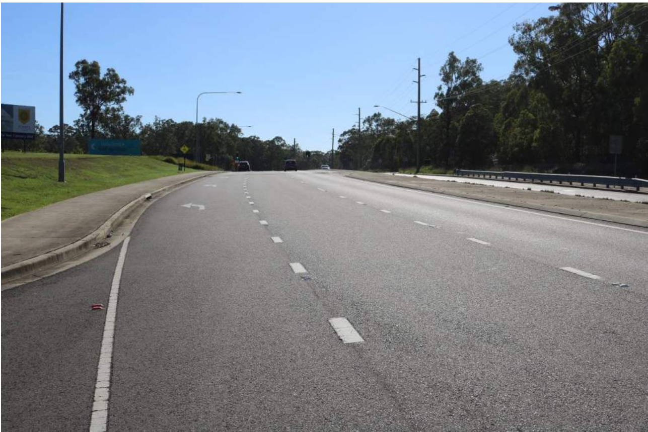
Photograph 3 – Raymond Terrace Road at Settler's Boulevard intersection
