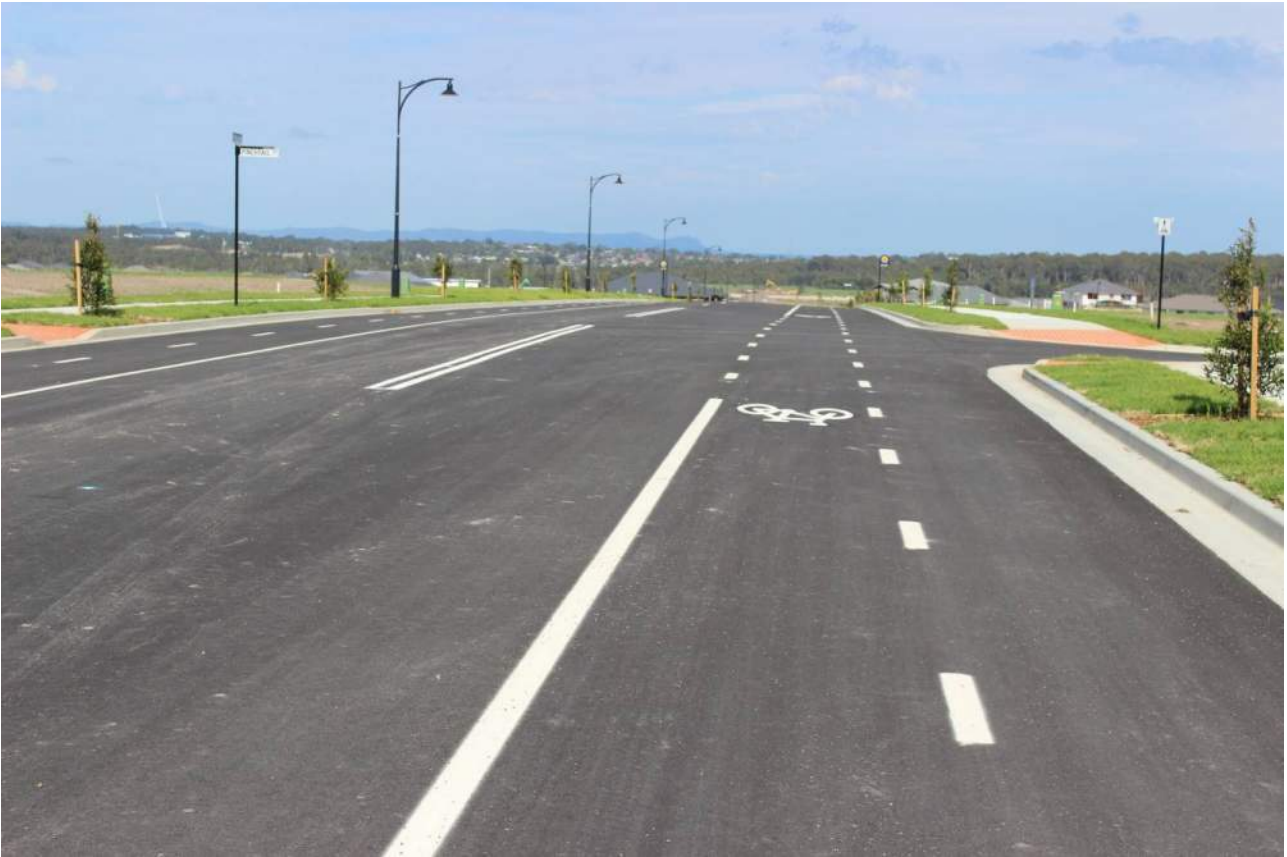
Photograph 4 – Dragonfly Drive near the site.
