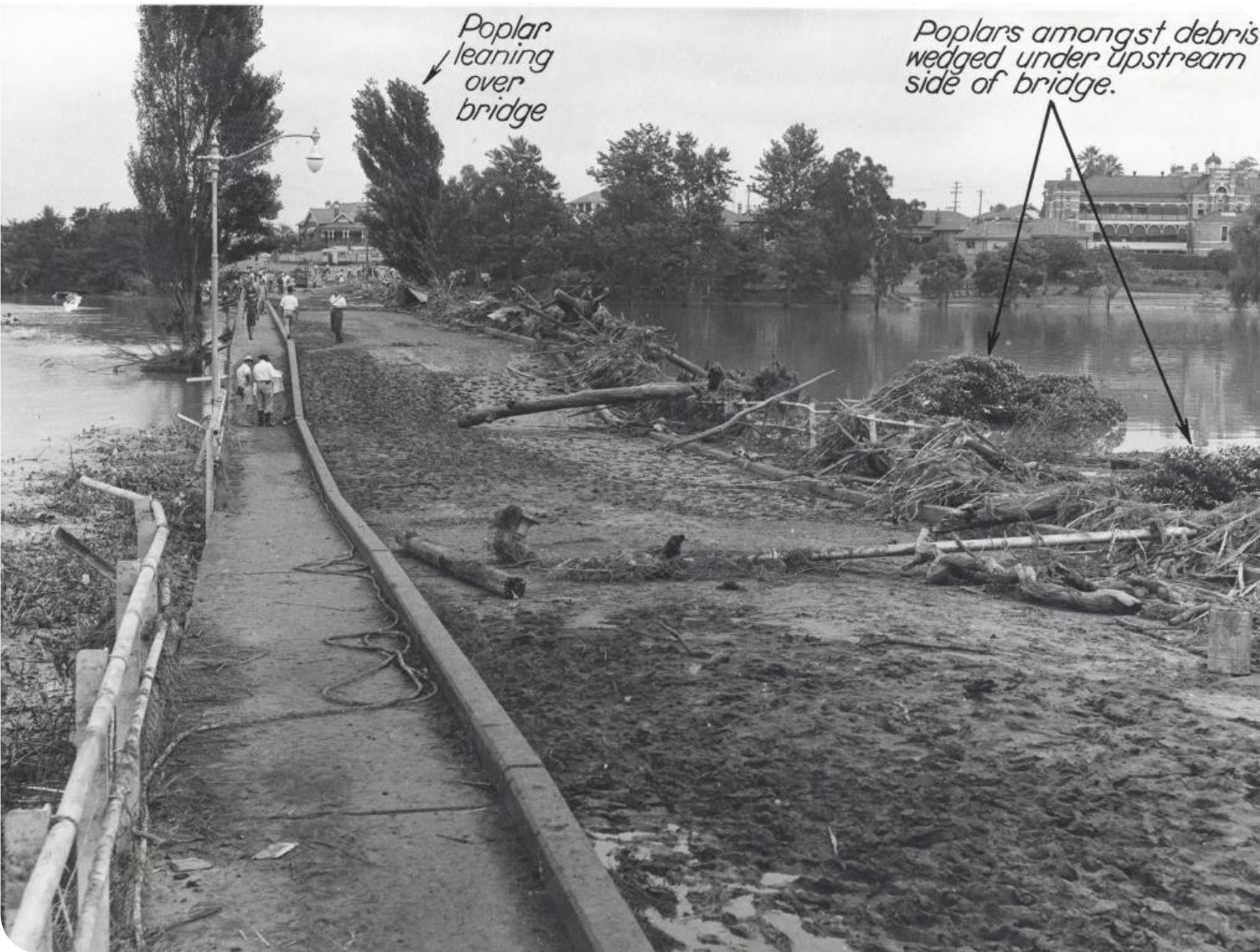
The collapsed Long Bridge 1955 flood.
