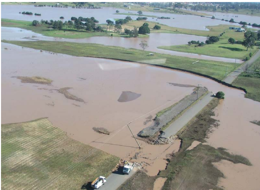
Photo 3: Failure of Oakhampton Road Control Embankment – June 2007
