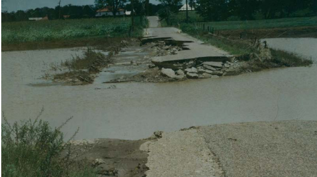
Photo 2: Failure of Oakhampton Road Control Embankment – March 1977
