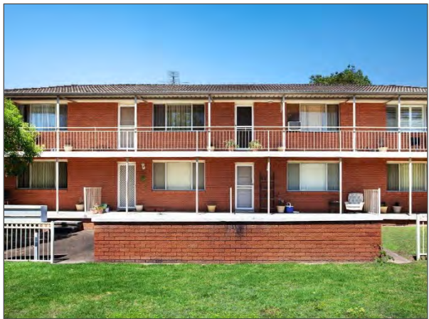
Established Low Rise Apartments in Telarah
