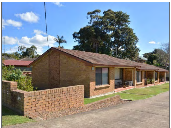
Established Medium Density Villas in East Maitland.
