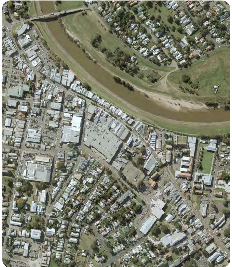
Central Maitland, Aerial View
