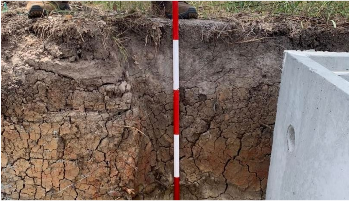
Plate 5. Trench along the in 5018 Raymond Terrace Road, with the only approximately 5cm of loam topsoils visible. (Source: Heritage Now 2021)
