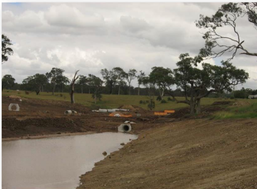
Figure 9: Channelisation and piping works need to address the natural characteristics of riparian areas and waterways in order to manage the interface between urban drainage systems and riparian areas downstream.
