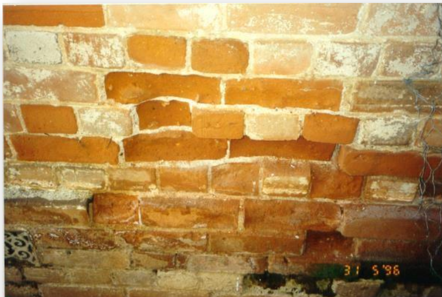
Rising damp and salt attack can lead to serious deterioration of masonry
