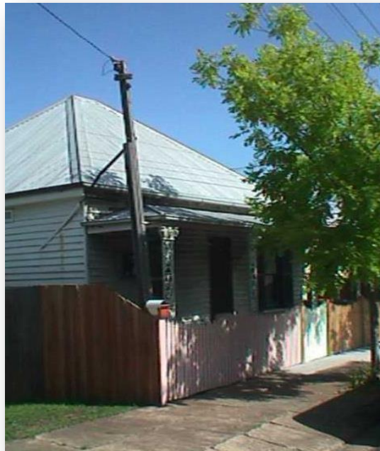
Alterations to this Victorian cottage returned the verandah to its original hipped form. A fence in keeping with the age of the building was also constructed
